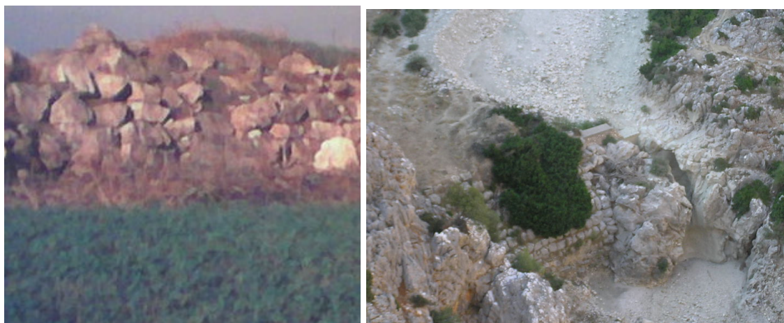
Fig. 5 (left) Cyclopean masonry of the Mycenaean dykes in Kopais, as preserved today; (right) The Alyzia Dam with its cyclopean masonry; the spillway is to the right of the dam wall.
