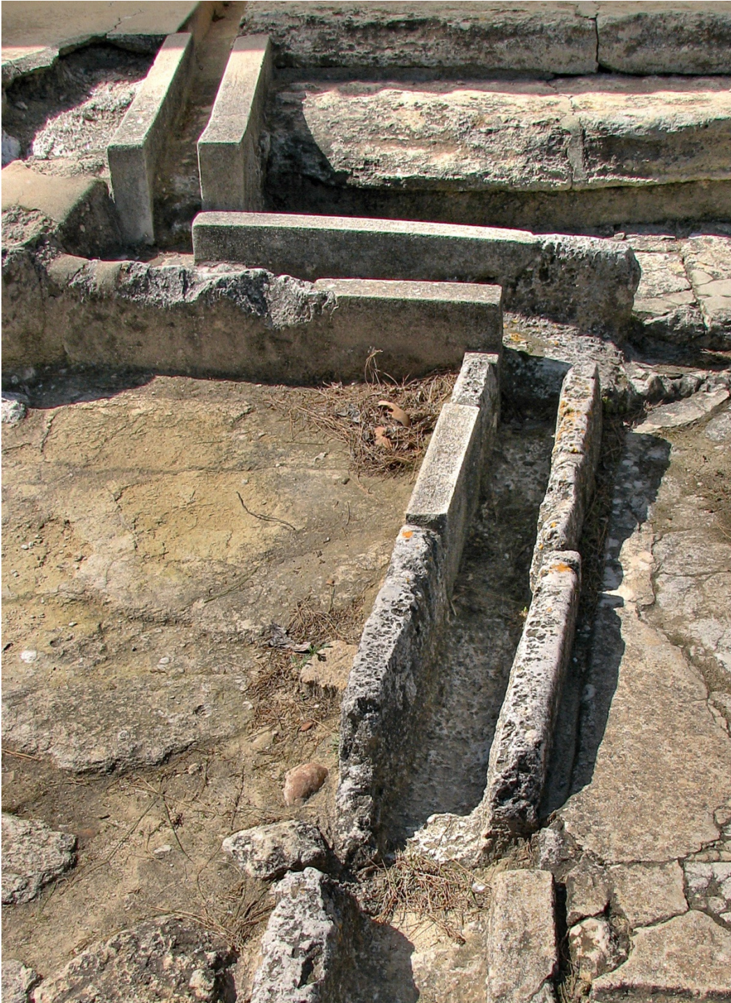
Carved stone elements of collecting rainfall falling from roof in Knossos
