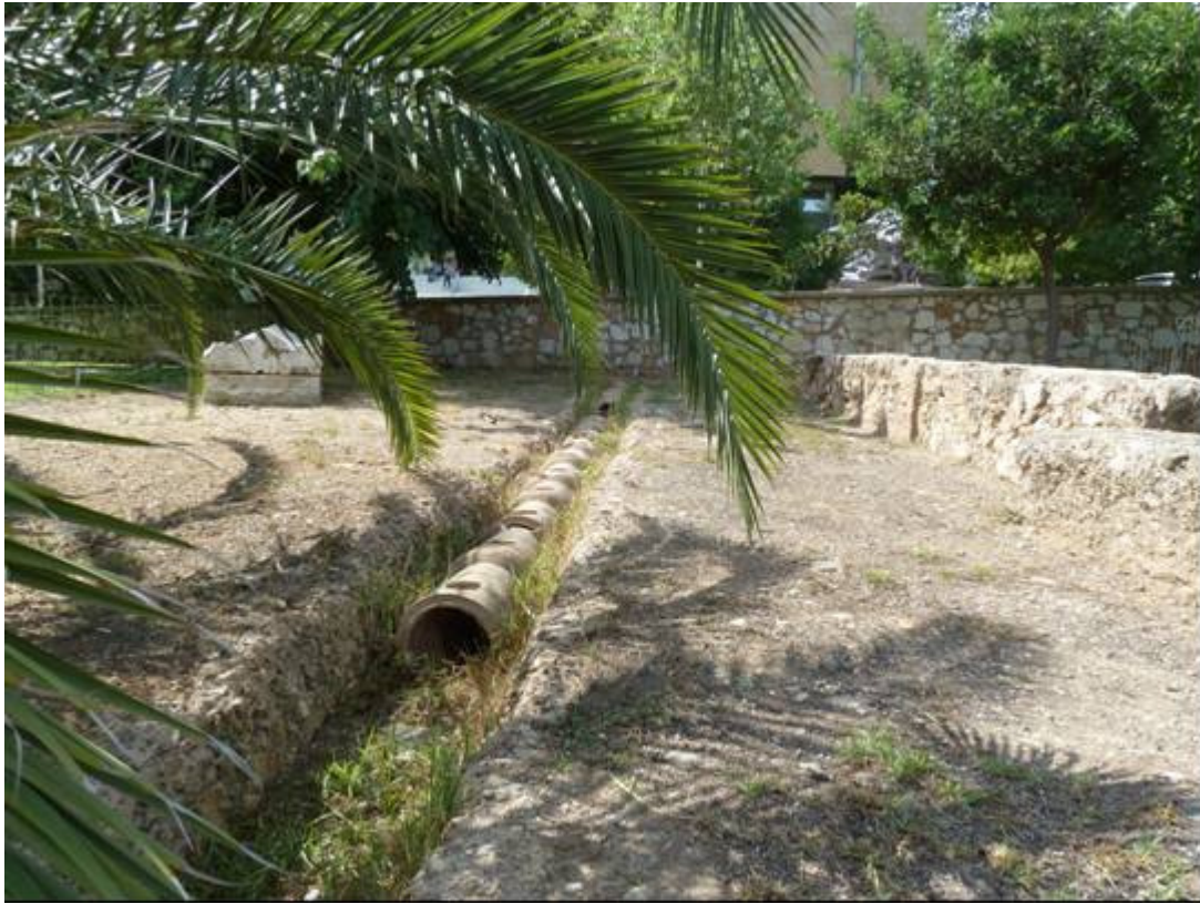
Figure 10.2. Terracotta pipes of the Peisistratean aqueduct in public display at Athens metro station of Evangelismos
