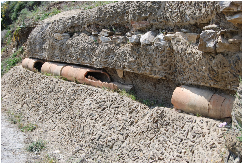
Figure 10.3. Naxos aqueduct, clay pipes
