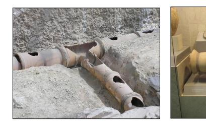
For cleaning and maintenance, in their upper part the pipes had elliptic openings covered by ceramic covers.
