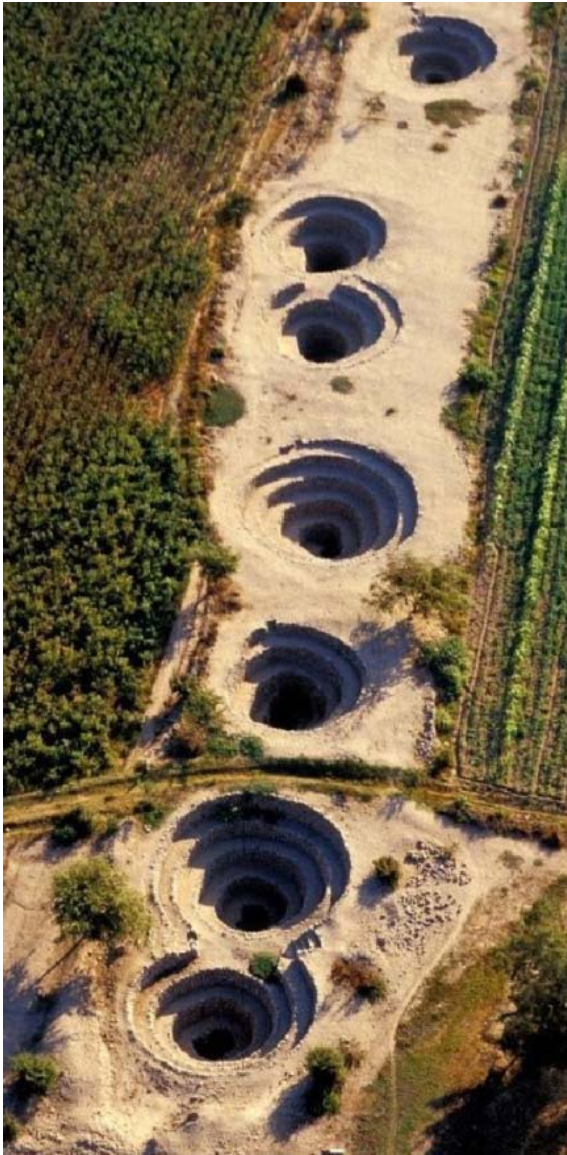
Openings along the Cantalillo aqueduct
