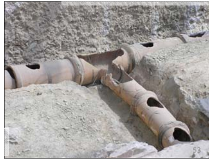
Part of the Peisistratean aqueduct and detail of the pipe sections and their connection (photos reproduced from newspaper Kathimerini).
