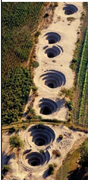
Openings along the Cantalillo aqueduct
