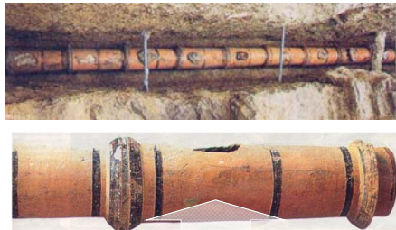
Part of the Peisistratean aqueduct and detail of the pipe sections and their connection (photos reproduced from newspaper Kathimerini).
