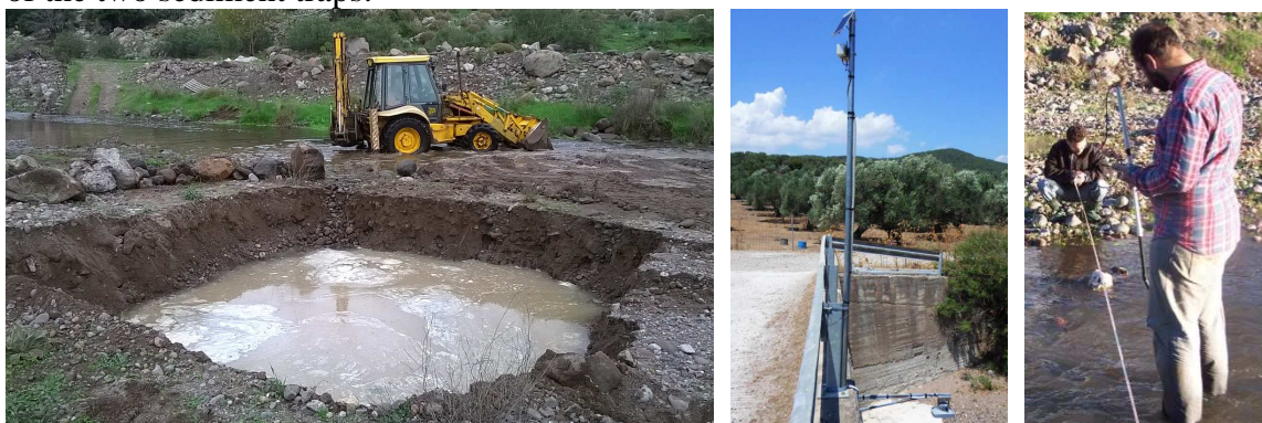
Figure 9. Sediment trap, level gauge and flow measurements in Tsiknias
