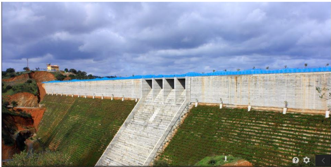
C. Photo of the downstream side of La Breña II dam from south
