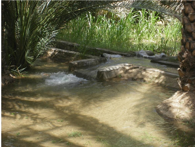
Figure 5. Outlet in a falaj system in Oman ( www.landolia.com ).
