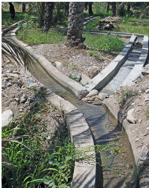
Figure 4. Diversion of water with stones in modern falaj system. (Source: yade.edu)
