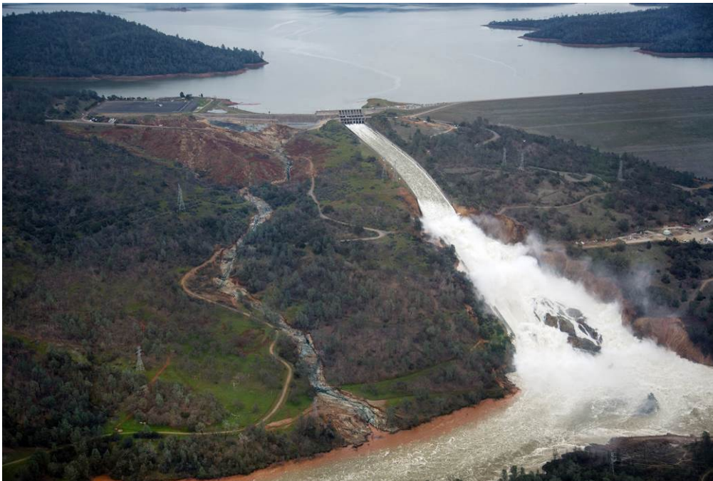
Image 28. February 15th, 2017. An aerial view of Oroville Dam's damaged spillways. Source: Dale Kolke, DWR.
