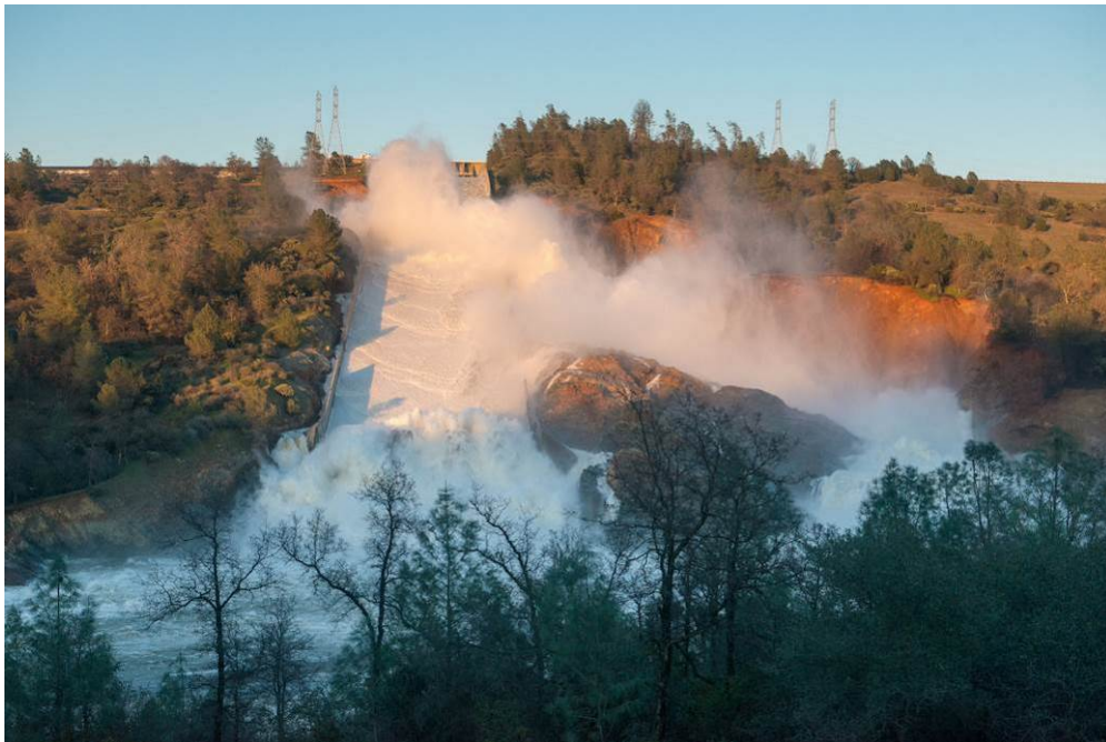
Image 26. February 11th, 2017. Water flowing over the damaged main spillway. Some of the discharge is flowing through the initial hole under the chute's left wall, creating a new channel. Source: Florence Low, DWR.
