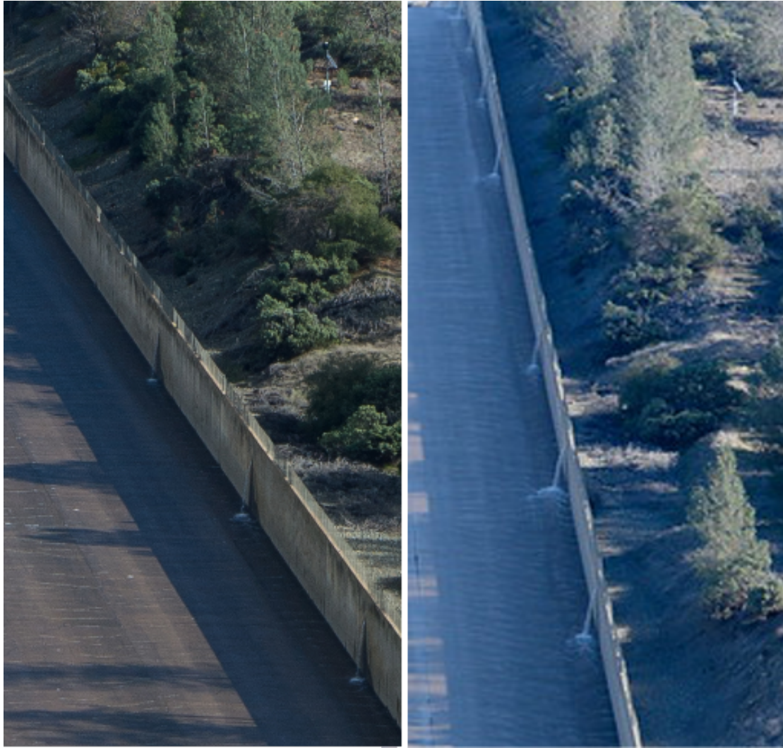
Image 39. Side by side comparison of drains in the spillway chute's left wall, left photo taken January 11, 2017 and right photo taken January 27, 2017. Sources: Kelly M. Grow, DWR and Bill Husa, Chico Enterprise-Record.
