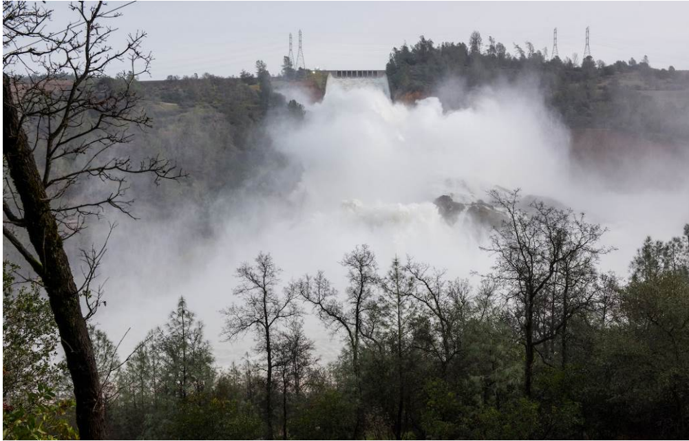
Image 27. February 13th, 2017. 2,830 m 3 /s (100,000 cfs) flowing over the main spillway. The chute's upper portion remains undamaged, but erosion quickly develops downstream. Source: Kelly M. Grow, DWR.
