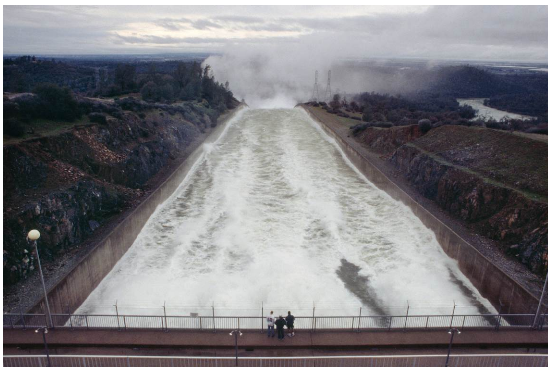
Image 11. January 2, 1997. Top view of Oroville Dam's main spillway. Discharge is 4,531 m 3 /s (160,000 cfs). Sources: Norm Hughes, DWR.
