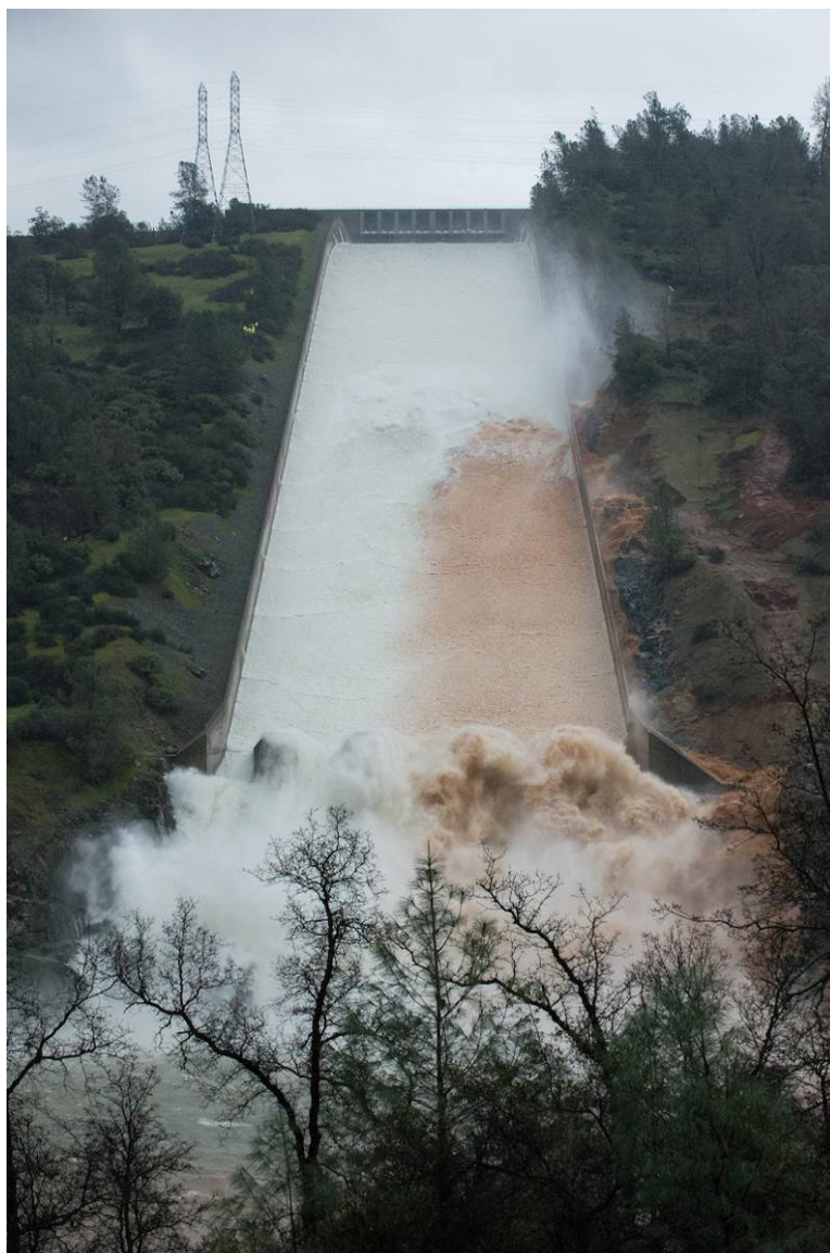
Image 16. February 8th, 2017. Discoloration of the flow along the Oroville Dam main spillway. Source: Kelly M. Grow, DWR.
