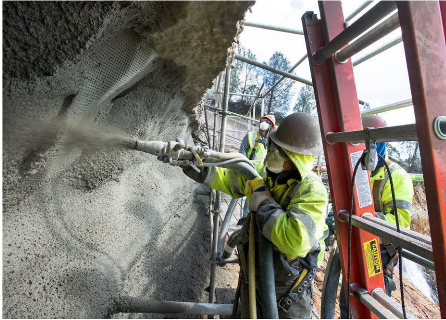
Image 31. March 5 th , 2017. Worker applies shotcrete under the main spillway chute's upper portion. Source: Kelly M. Grow, DWR.
