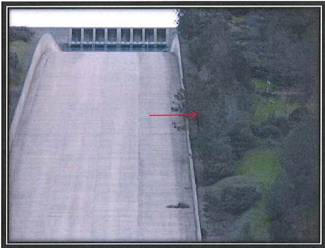
Image 15. August 3, 2015. A "lone tree" along the left wall of the Oroville Dam main spillway. Source: Division of Dam Safety, DWR.
