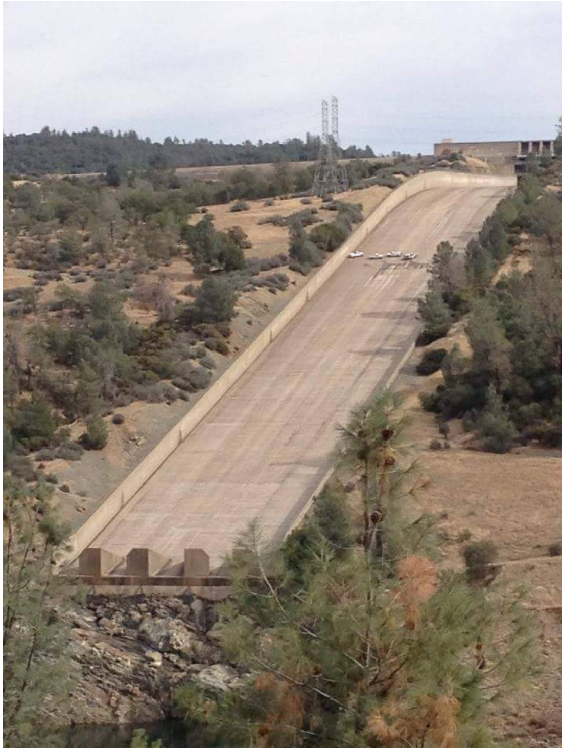
Image 14. 2013 image showing repairs being made on the Oroville main spillway chute. Source: Unknown, possibly DWR.
