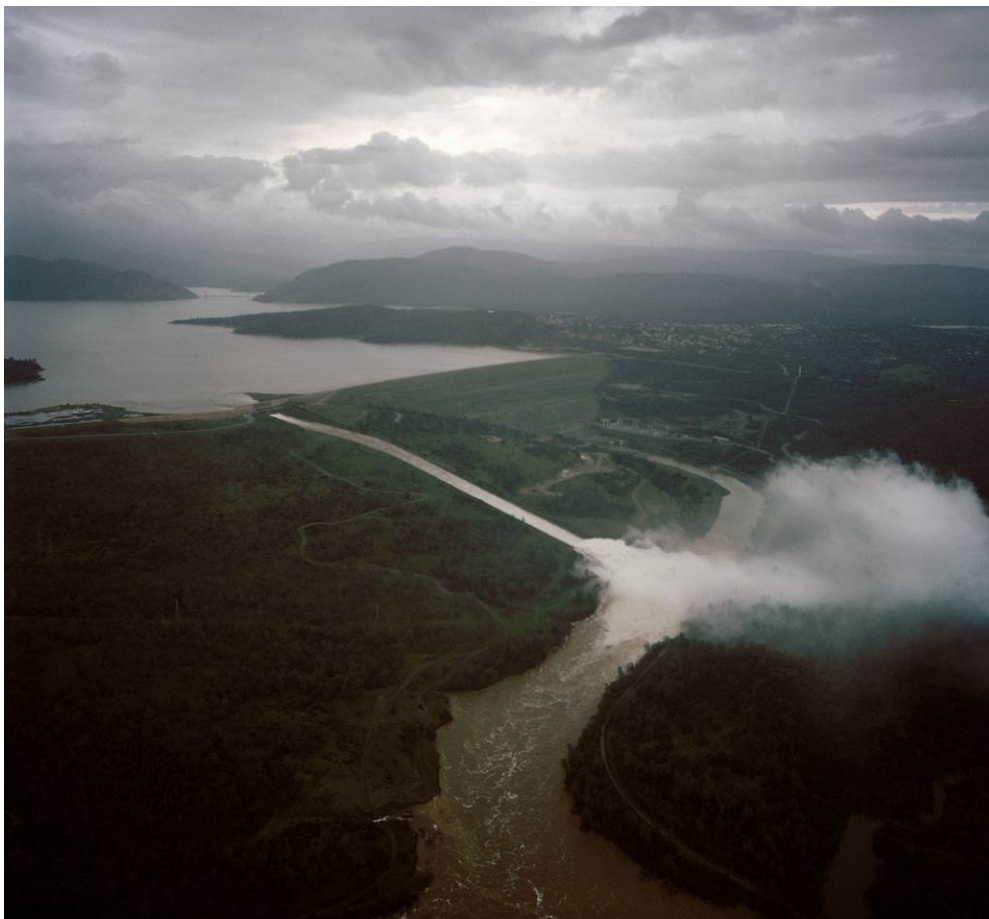
Image 8. February 21, 1986. The Oroville Dam main spillway operating at the maximum scheduled discharge of 4,250 m 3 /s (150,000 cfs). Source: Norm Hughes, DWR.
