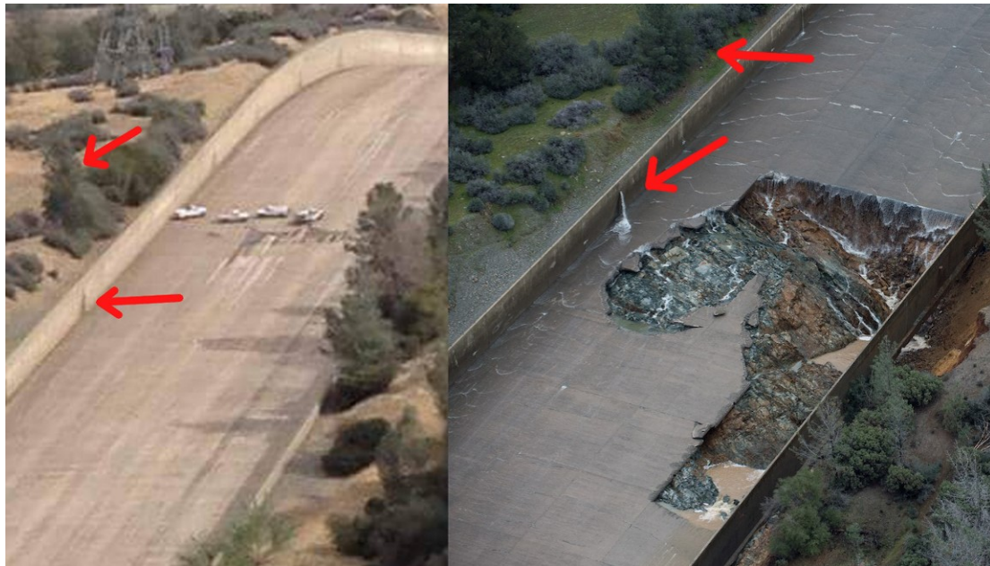
Image 37. Comparison of 2013 chute repairs and February 6th, 2017 initial chute damage. Sources: Unknown and Kelly M.Grow, DWR.
