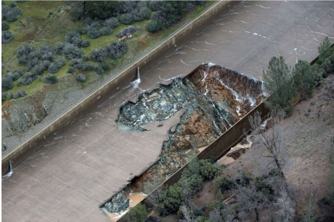
Image 40. February 7th, 2017. Side view of the initial spillway chute failure. Source: Kelly M. Grow, DWR.
