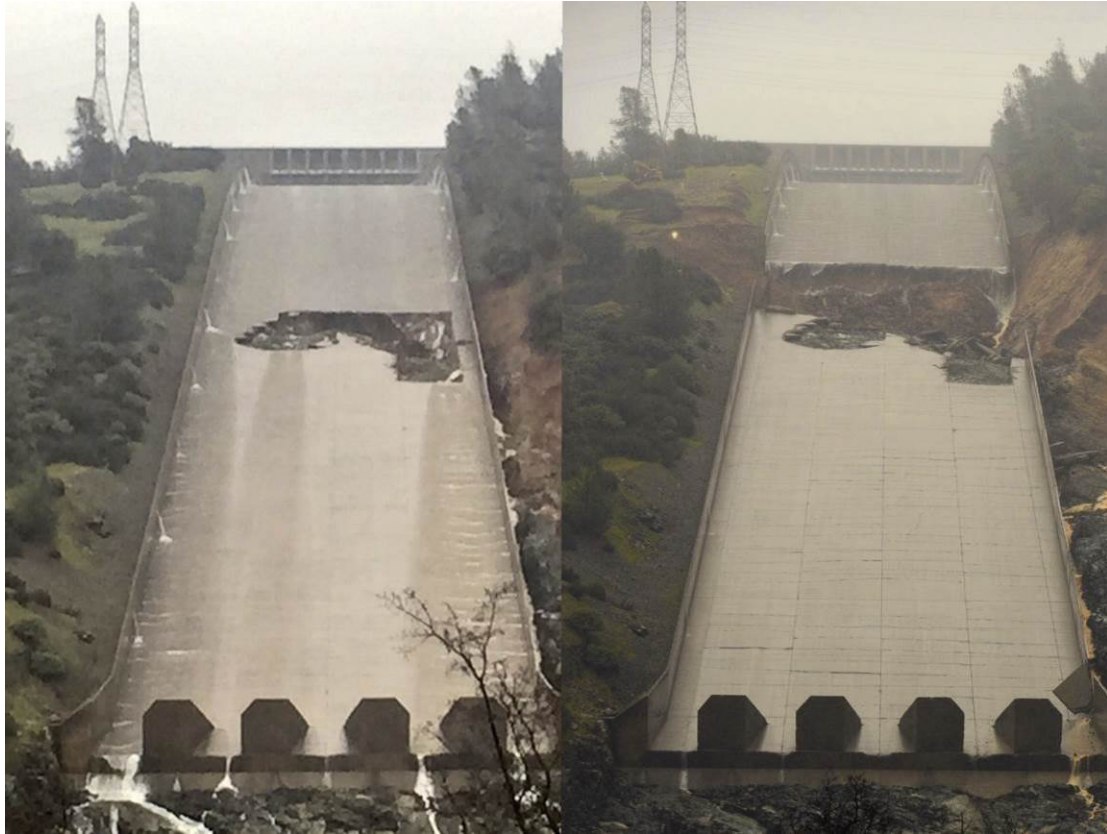
Image 19. Comparison of the February 7 main spillway hole (left) to the damage on February 9 (right). The erosion appears to be moving uphill. Sources: Kelly M. Grow, DWR and the Metabunk.org forum.
