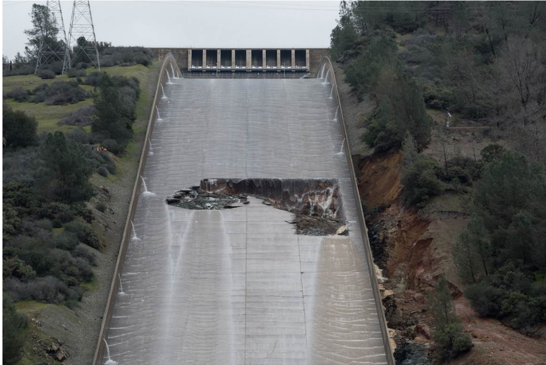
Image 17. February 7 th , 2017. Front view of the initial main spillway chute damage. Source: Kelly M. Grow, DWR.
