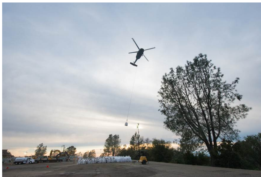
Image 29. A helicopter transports a bag of large rocks over to the emergency spillway. Source: Florence Low, DWR.
