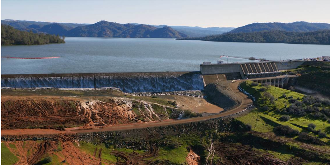
Image 21. February 11, 2017. Water flows over the Oroville Dam emergency spillway for the first time. Source: Zack Cunningham, DWR.
