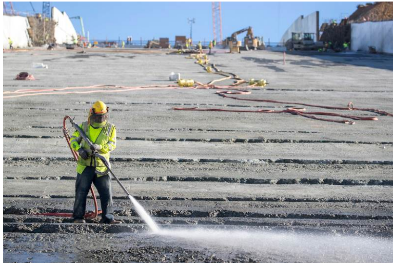
Image 41. October 25, 2017. A worker uses water and compressed air to clear the concrete floor of the new Oroville Dam spillway chute, in preparation for a new layer of RCC. The new structure is nearly complete.
