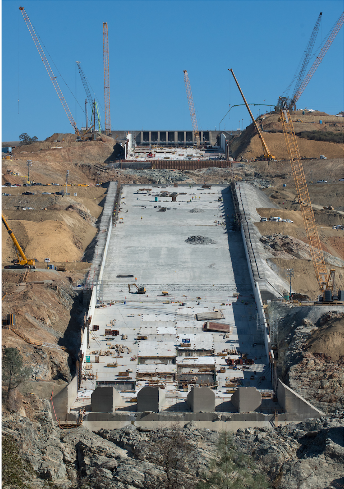
Image 33. October 13th, 2017. View of the Oroville Dam main spillway chute repair work. Source: Kelly M. Grow, DWR.
