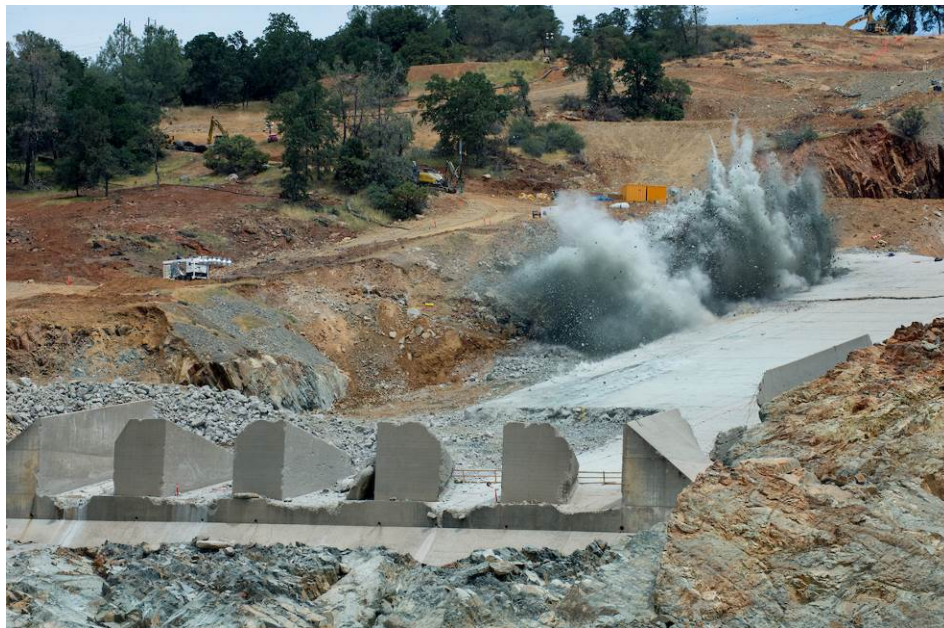
Image 32. May 30 th , 2017. Blasting is used at the lower portion of the main spillway chute. Source: Kelly M. Grow, DWR.
