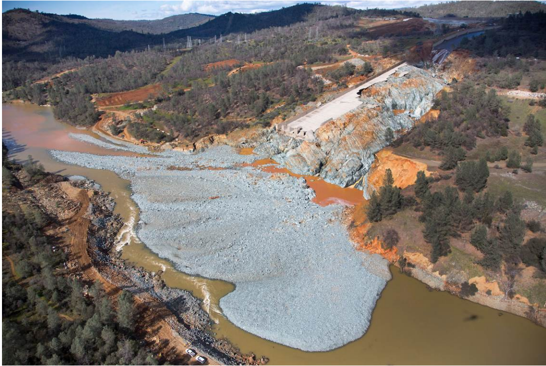
Image 30. February 27th, 2017. Aerial view of the Oroville Dam main spillway. Large sections have eroded away and ended up in the Feather River as debris. Source: Dale Kolke, DWR.
