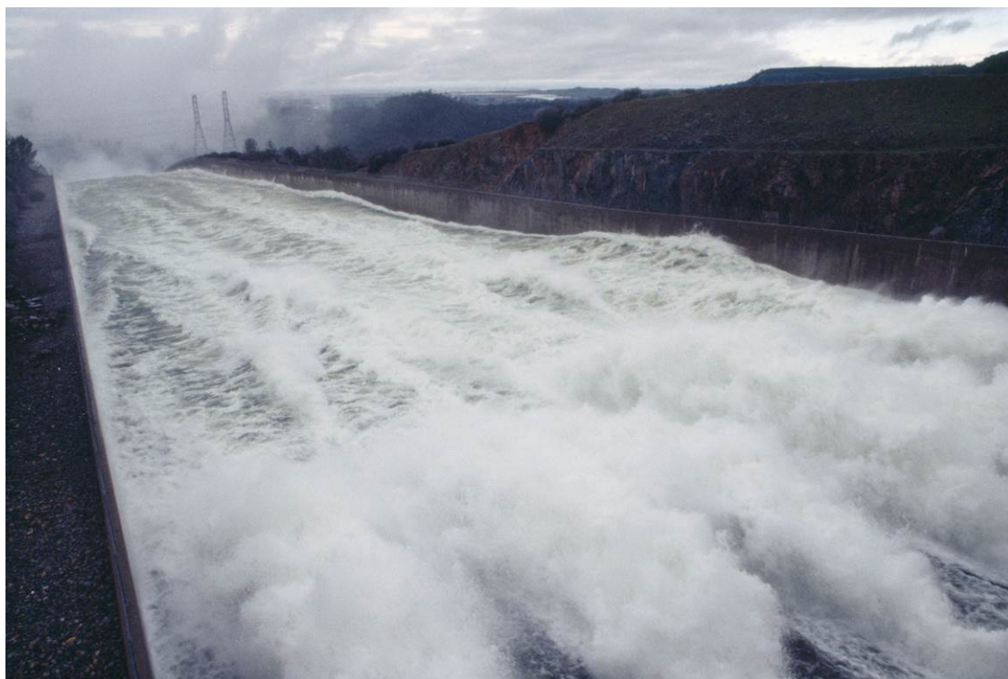
Image 10. January 2, 1997. Side view of Oroville Dam's flood control outlet, as releases reach 4,531 m 3 /s (160,000 cfs) for the first time in history. Sources: Norm Hughes, DWR.
