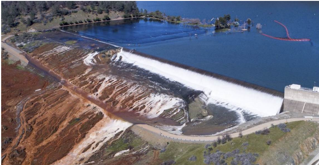
Image 22. February 11, 2017. Image of the flooded parking lot and access road located next to the emergency spillway. Source: Metabunk.org
