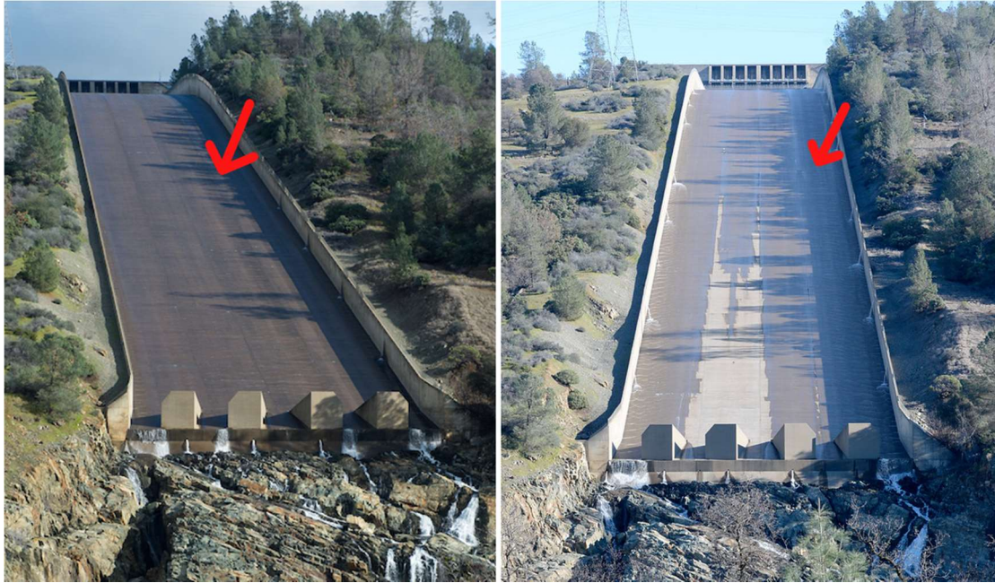
Image 38. Views of the Oroville Dam main spillway chute. Left photo taken January 11th, 2017, and right photo taken January 27th, 2017. A red arrow points to the location of the initial chute failure. Sources: Kelly M. Grow, DWR and Bill Husa, Chico Enterprise-Record.
