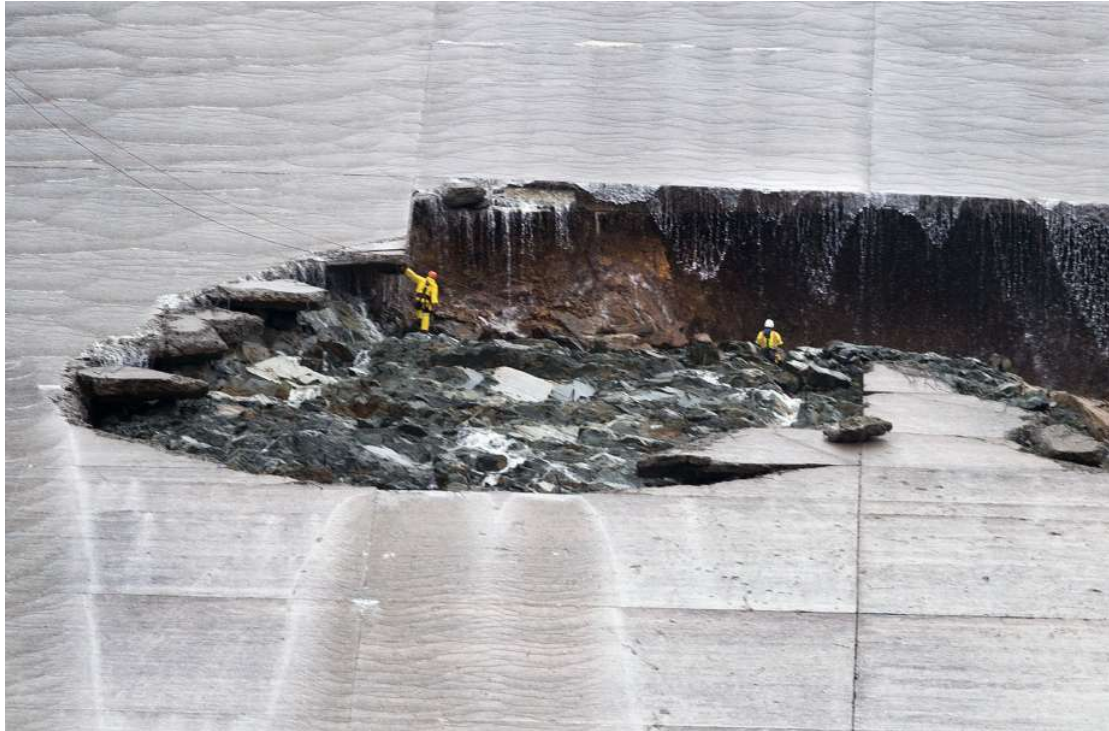
Image 18. February 7, 2017. Workers examining the ruptured Oroville Dam main spillway. Source: DWR.
