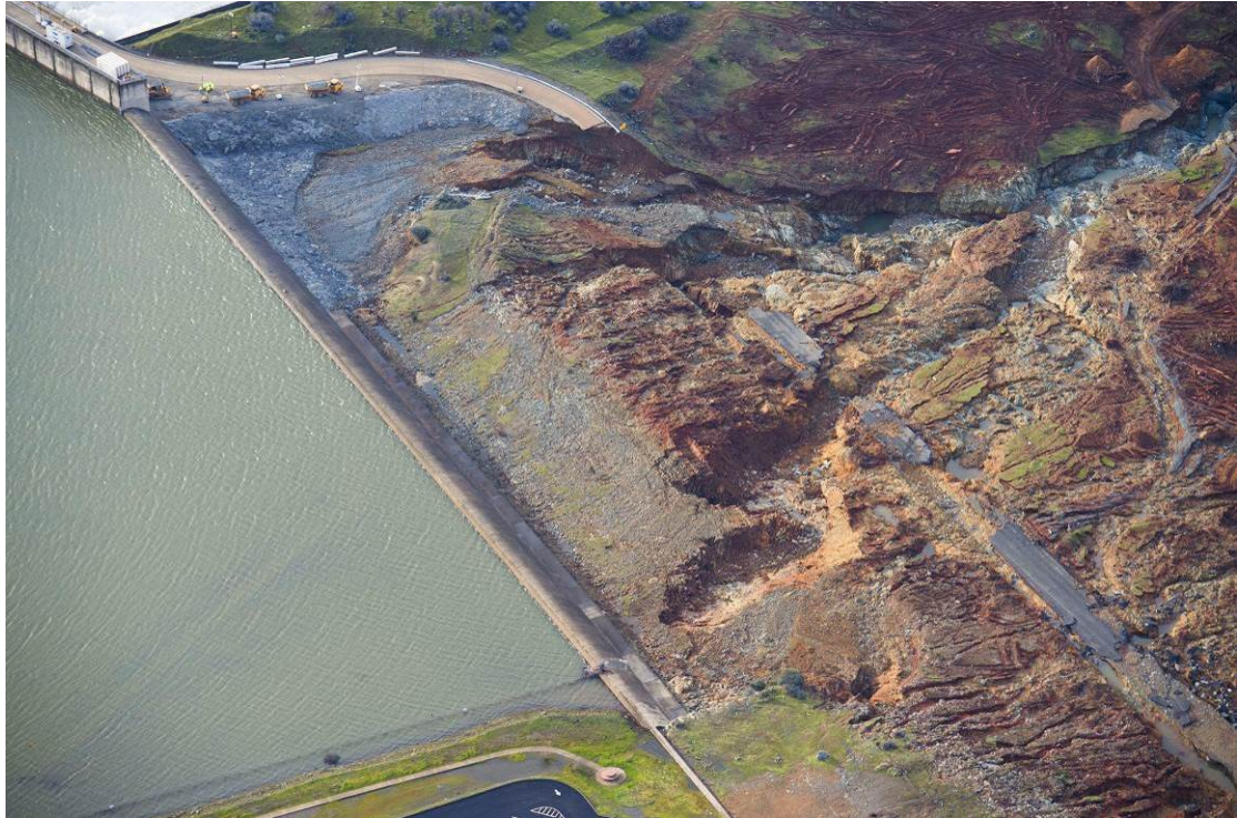
Image 23. February 13, 2017. The aftermath of the erosion caused by flows over the emergency spillway. Source: Randy Pench, Sacramento Bee.
