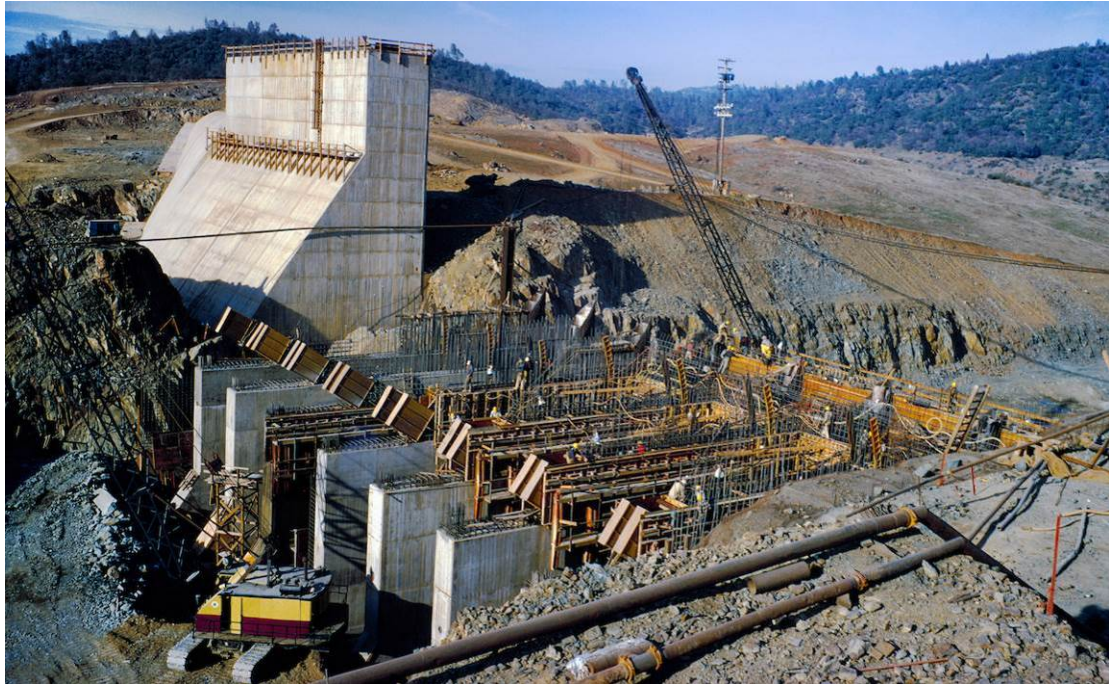
Image 7. Construction of the Oroville Dam main spillway flood control outlet. Photo taken January 1967. Source: DWR
