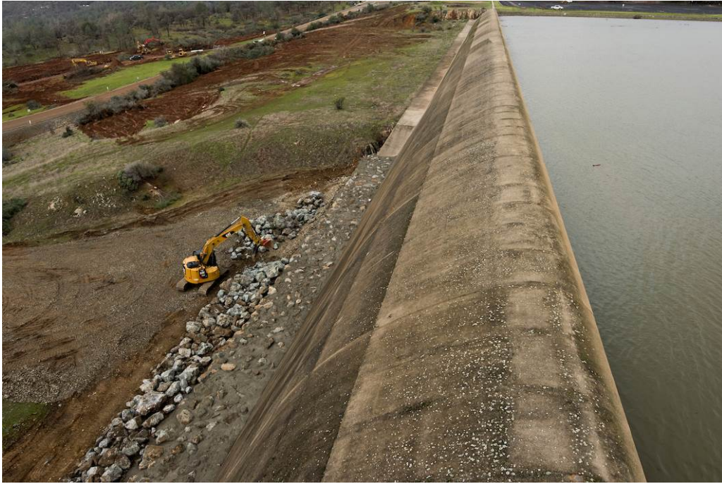
Image 20. February 10th, 2017. Workers prepare the emergency spillway for use by placing large rocks at its foot. Source: Brian Baer, DWR.
