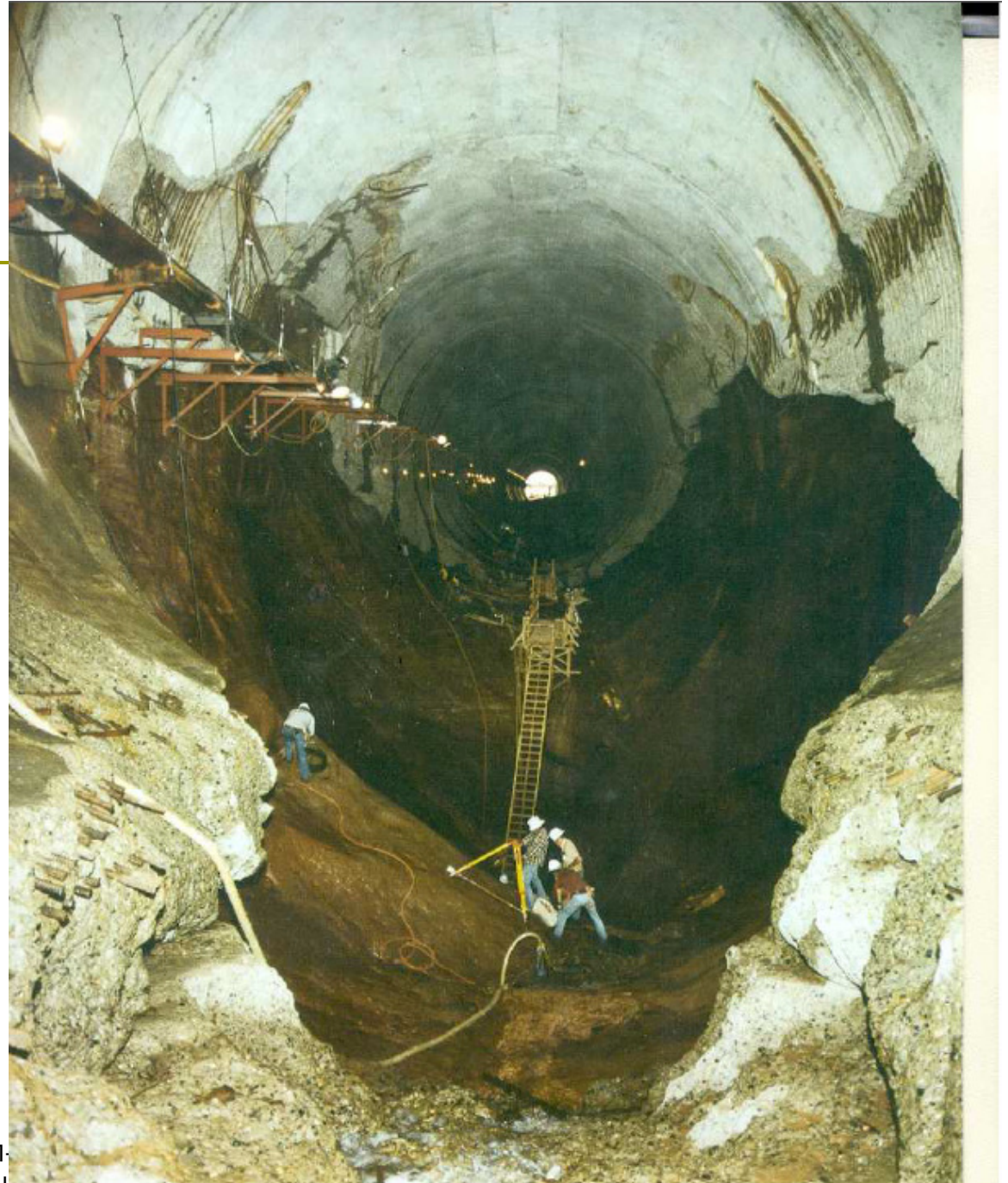
FRONTSPICE--Glen Canyon Dam. Left Spillway Tunnel Sept. 1983. The "big hole" in the spillway invert was 11 meters deep. Photo C557-400-690NA
