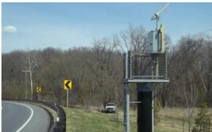
Figure 8.4 Monocacy River at Bridgeport Station.
