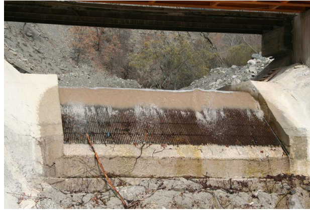
Trash rack of water intake
