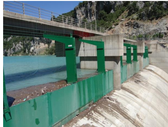
Spillway and fusegates
