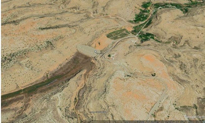
The upper (Al-Bilad) dam in Wadi Derna, as shown on Google Earth. Image from June 2023.
