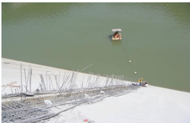
Figure 4b. Damage to vertical joint of Zipingpu CFRD caused by the 2008 Wenchuan earthquake in China (4a) and the repair of a damaged vertical joint (4b). During the earthquake the reservoir volume was about 30% of that due to normal water level (photos courtesy Xu Zeping)
