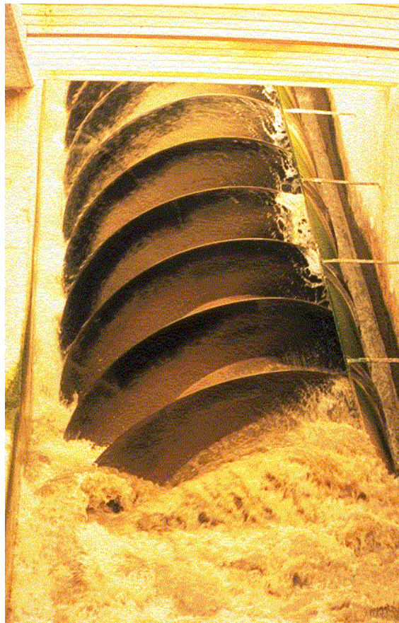
Figure 2. Archimedes's water screw in its modern form, as implemented in the wastewater treatment plant of Athens (one of 5 screws that pump 1 million m 3 per day).
