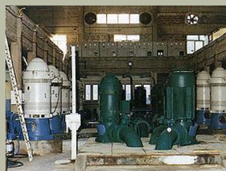
Kiourka pumping station
