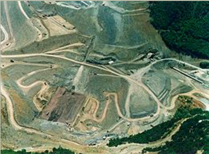
Evinos dam during construction
