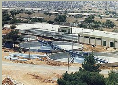
Aspropyrgos water treatment plant
