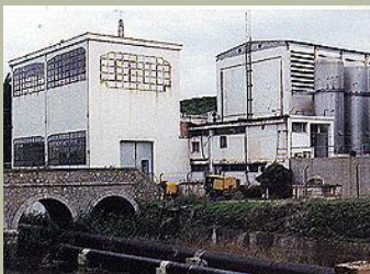
Hylike, main pumping station
