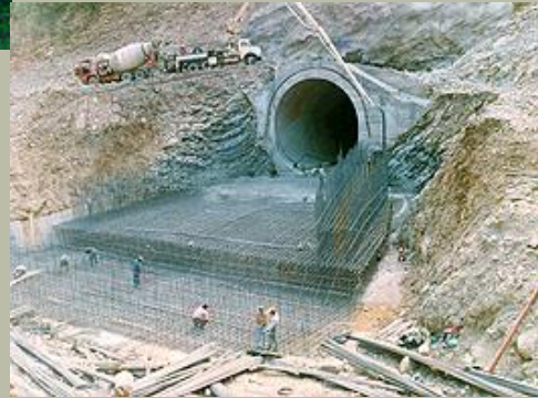
Construction of the Evinos-Mornos connection tunnel
