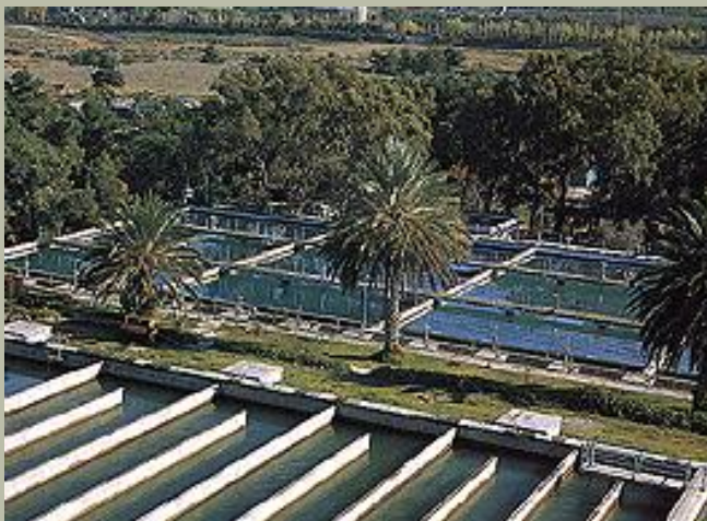
Perissos water treatment plant
