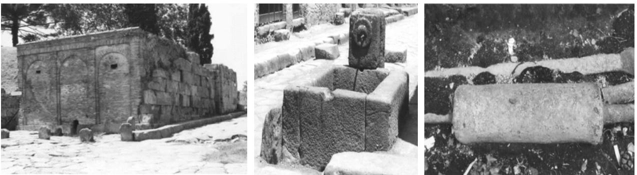
Figure 9 Elements of water supply system at Pompeii: (left) castellum divisorium at Porta Vesuvii housed in the large brick building; (middle) public fountain; and (right) lead pipe with enlarged section of junction box.
