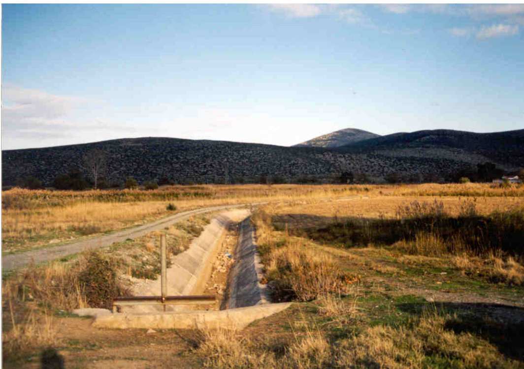
Photo 9: Irrigation canal taking water from the Mauroneri stream through a wear, a bit before the homonymous springs.
