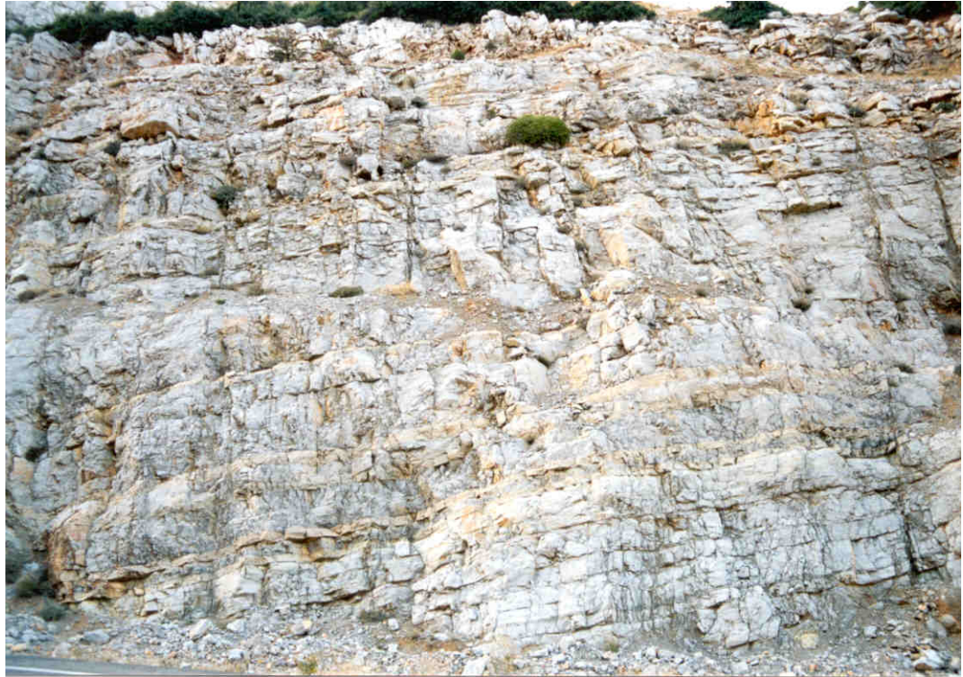
Photo 11: Precipitate front of karstic limestone in the area of Mavroneri springs. The limestones are developed in horizontal and precipitate layers and they are extremely broken.
