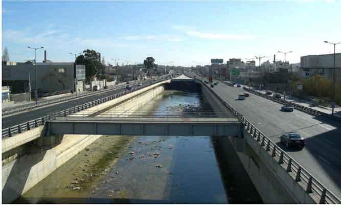
*Fig. 5: Combination of the drainage channel with Kephisos Avenue (Source: Laskaris 2008)*
