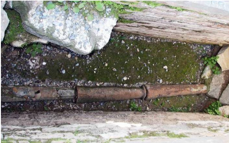
Terracotta pipe sections (Buffet and Evrard, 1950)
