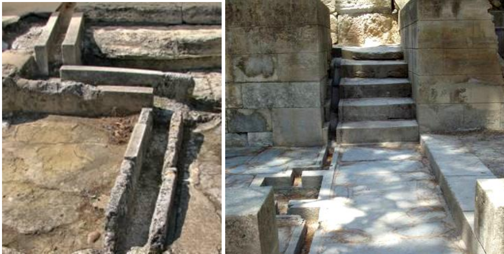
Figure 1. Minoan rainwater collection systems in the Knossos palace: carved stone elements of a conduit for the flow of rainwater falling on the roof (left) and part of restored stairway with parabolic runnels for rainwater flow (right); photos by A. Angelakis.
