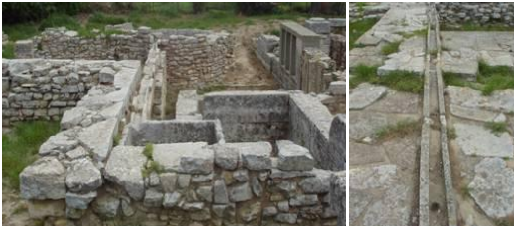
Figure 2. Minoan stone conduit systems (part of aqueduct) at Tylissos: to transfer the water from a sedimentation tank to the main storage cistern (left) and part of distribution network (right); photos by A. Angelakis.
