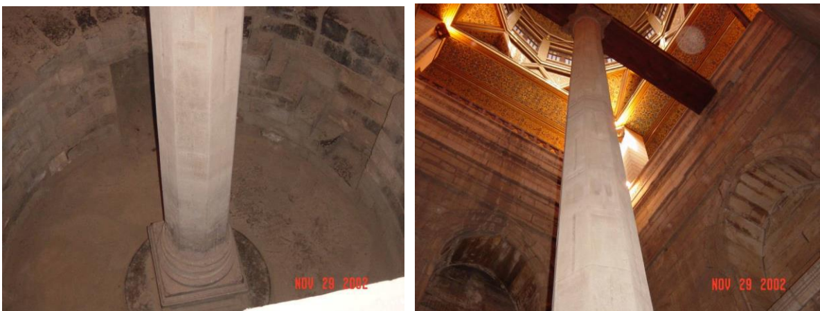
Fig. 8 The Roda Nilometer, near Cairo, as it stands today; water entered and filled the Nilometer chamber up to river level through three tunnels (Credit: Aris Georgakakos).
