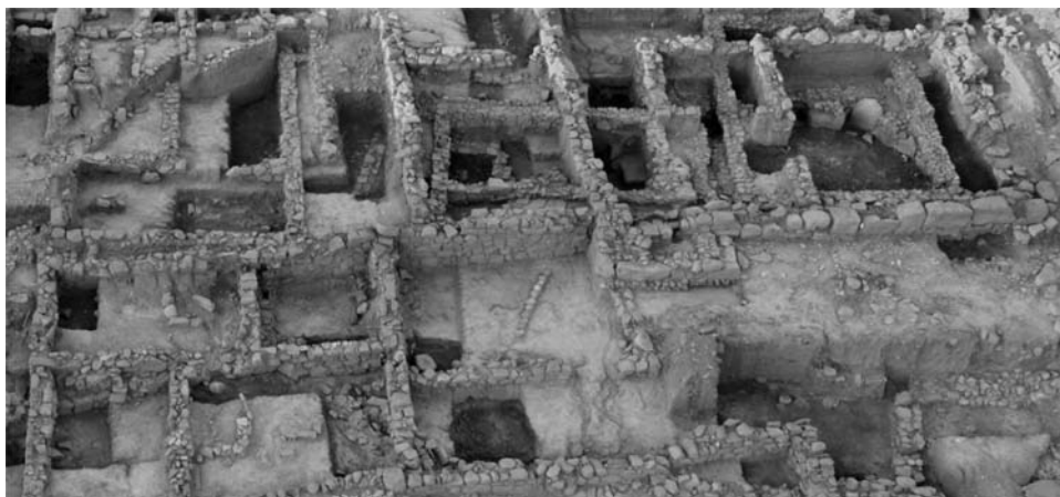
Figure 7 | The central area of the settlement with various phases/layers of the buildings.
