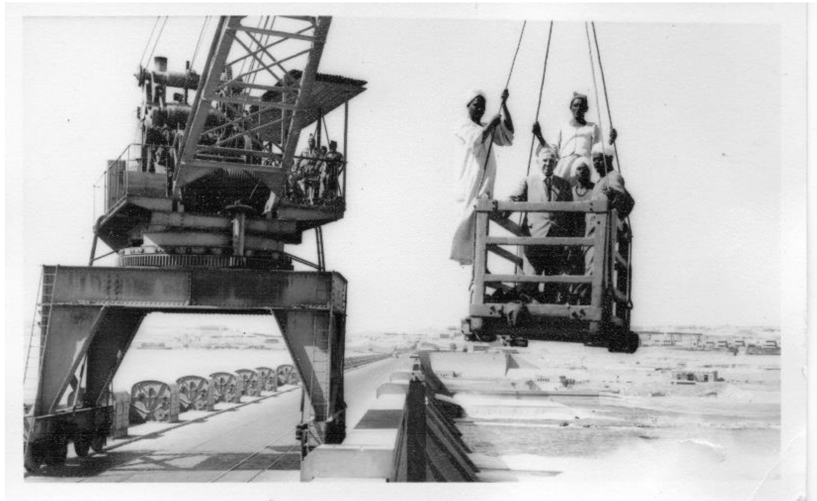
Inspection Aswan Dam
