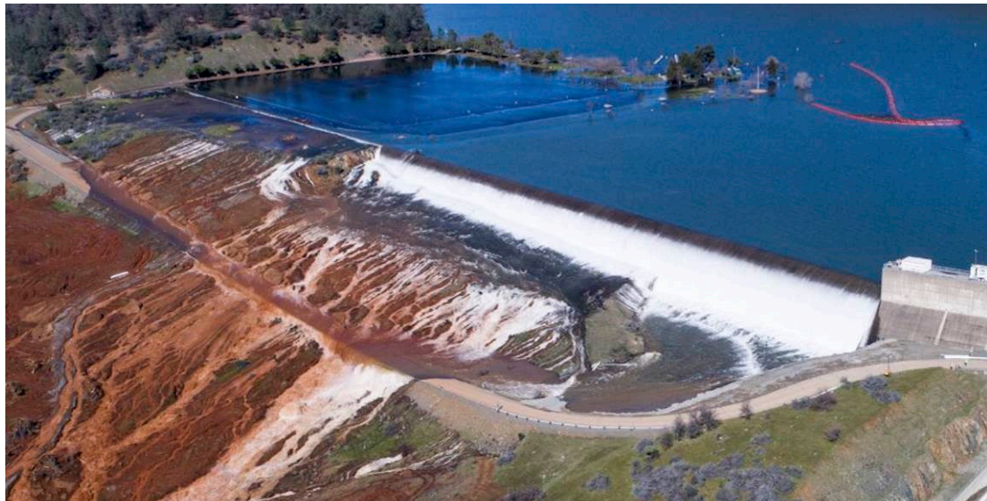
Figure 3. 11 February 2017. Image of the flooded parking lot and access road located next to the emergency spillway [39].
