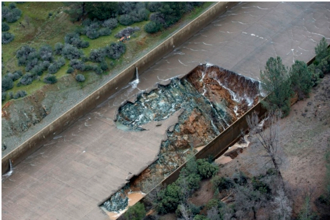
Figure 7. 7 February 2017. Side view of the initial spillway chute failure [38].
