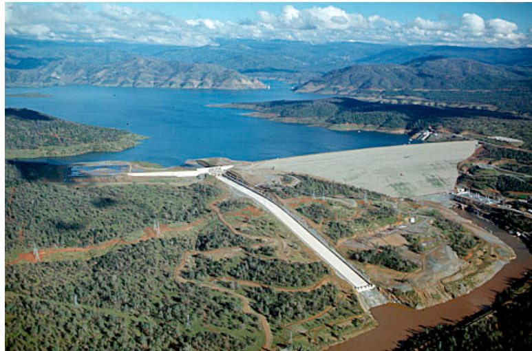
Figure 1. Aerial view of Oroville Dam [26].
