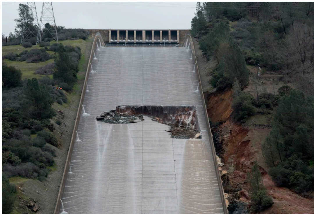
Figure 2. 7 February 2017. Front view of the initial main spillway chute damage [38].
