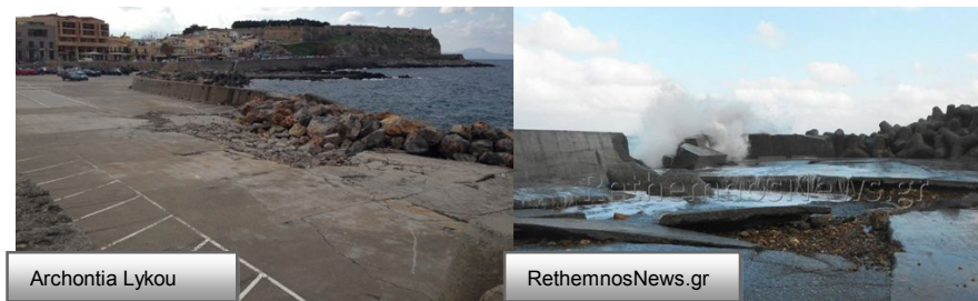
Figure 4: Damages of the base of windward wave breakwater (a) previous damages, photograph taken on January 4 th , 2014, (b) new damages after structural repairs, photograph taken on January 14 th , 2015
