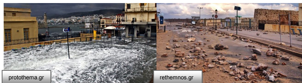
Figure 5: Penetration of seawater through overtopping to the wider area of port facilities and debris from the windward wave breakwater damages
