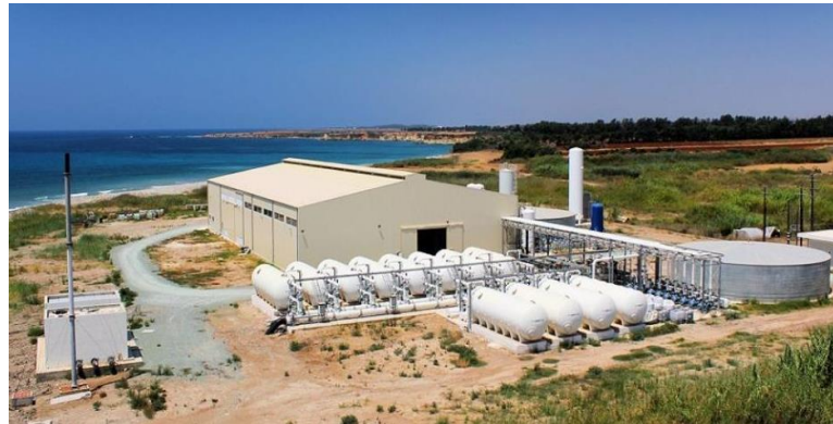
Desalination Plant, Pafos, Cyprus [7]
