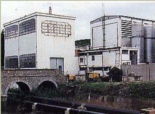
Yliki, main pumping station
