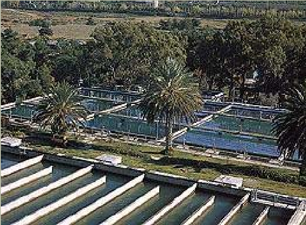
← Perissos water treatment plant
