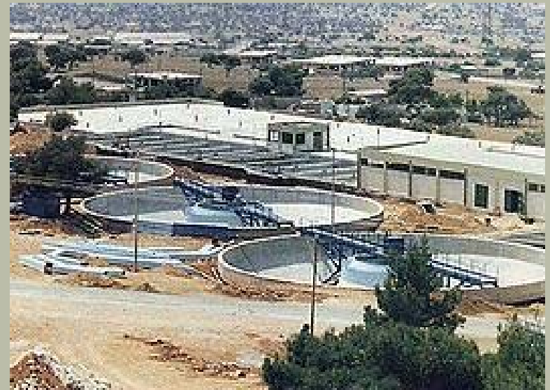
Aspropyrgos water treatment plant →
