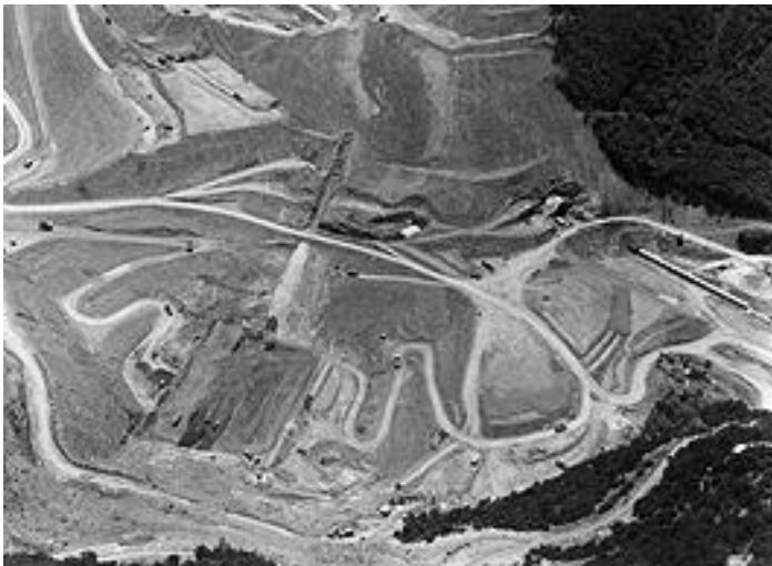
Evinos dam during construction
