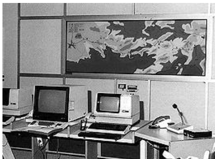
Aqueduct supervising & control centre
