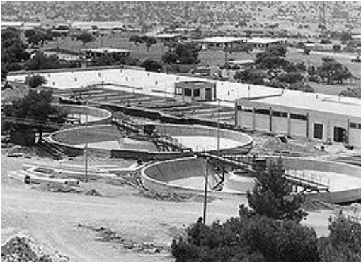
Aspropyrgos water treatment plant →
