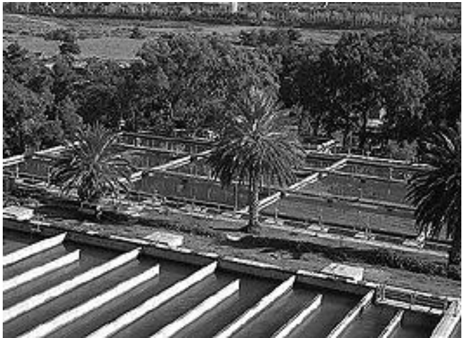
← Perissos water treatment plant
