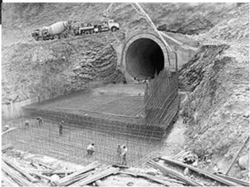
Construction of the Evinos-Mornos connection tunnel
