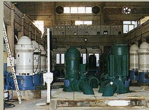
Kiourka pumping station
