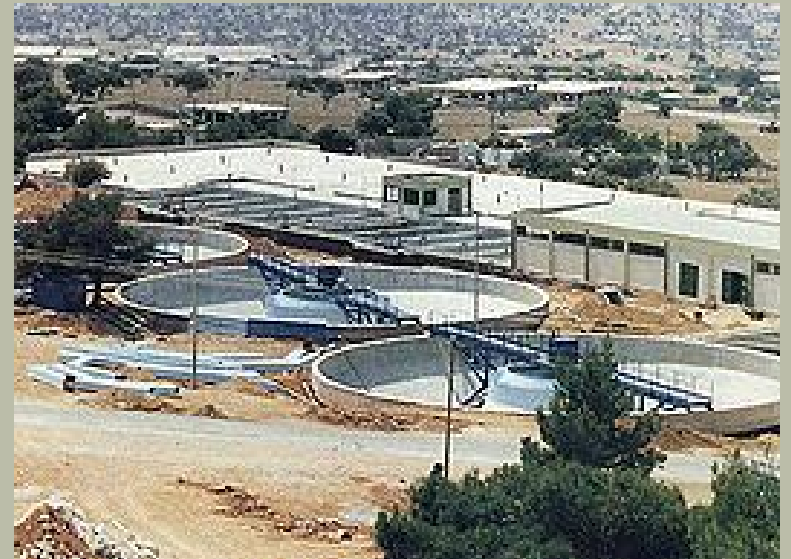
Aspropyrgos water treatment plant →
