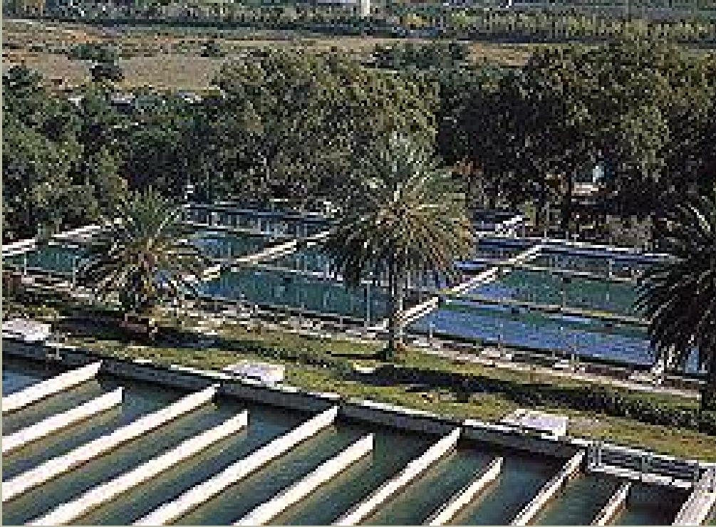
← Perissos water treatment plant
