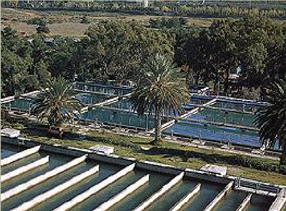
Perissos water treatment plant
