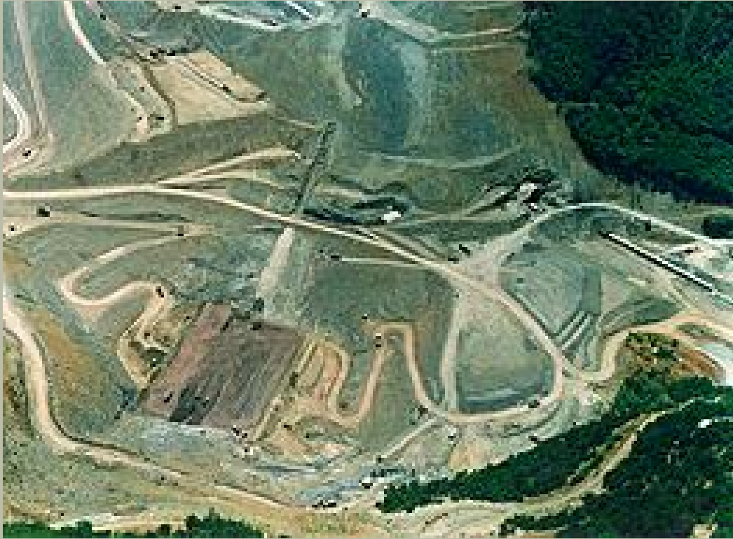
Evinos dam during construction
