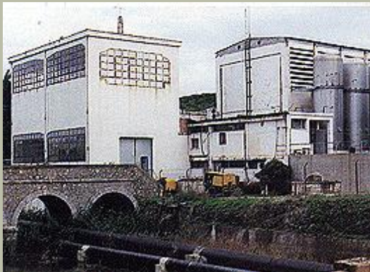
Hylike, main pumping station
