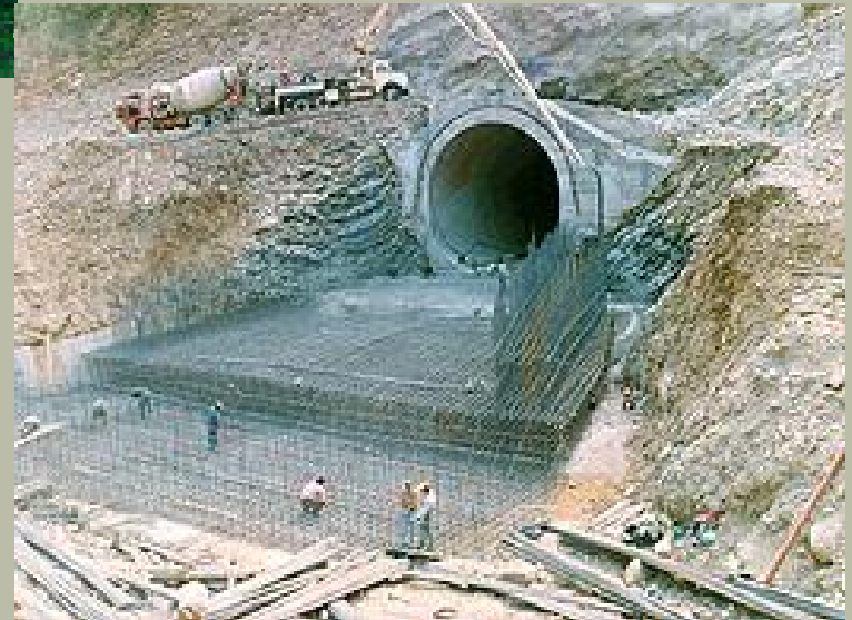
Construction of the Evinos-Mornos connection tunnel
