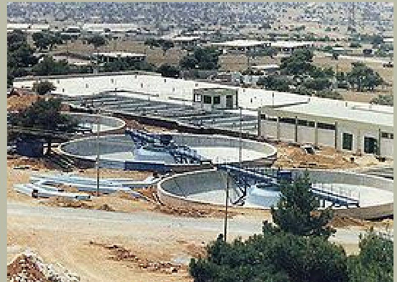
Aspropyrgos water treatment plant
