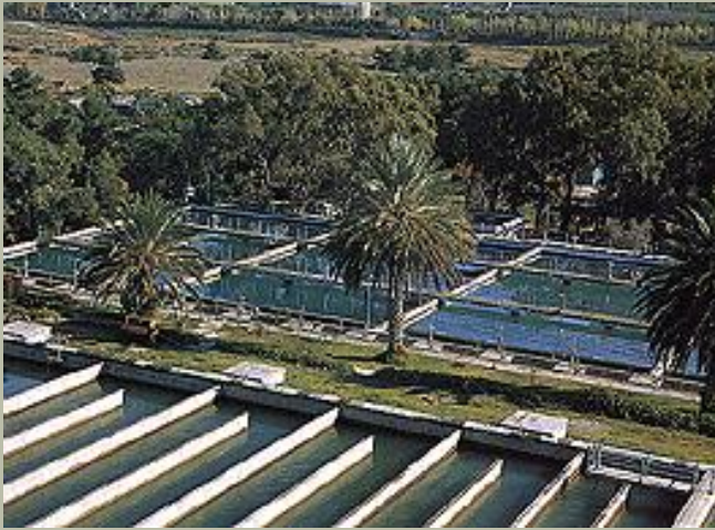
Perissos water treatment plant
