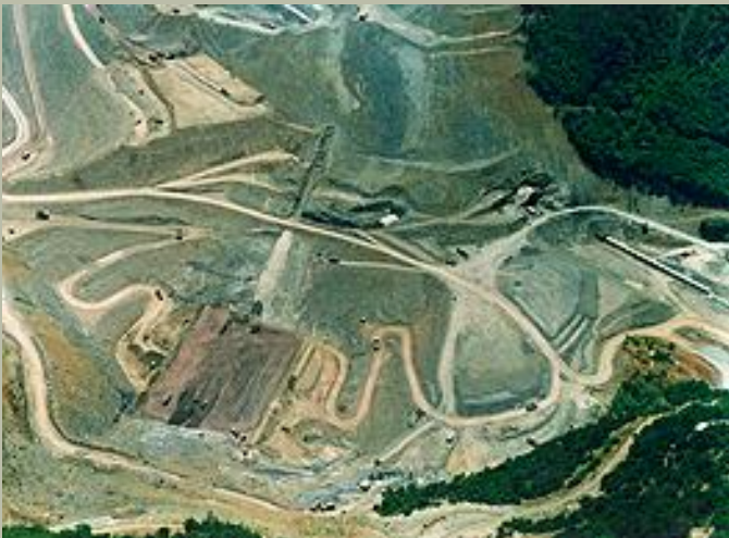
Evinos dam during construction
