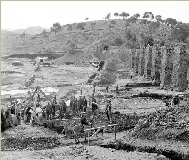
Restoration of the Hadrianean aqueduct (19 th century)
