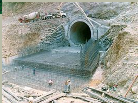
Construction of the Evinos-Mornos connection tunnel
