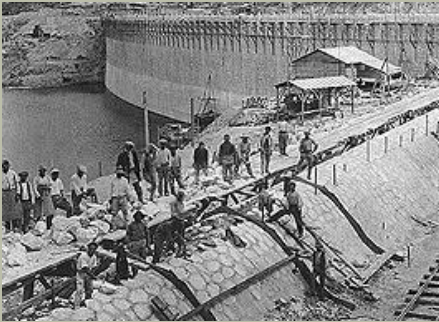
Construction of spillway, 1928
