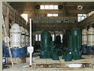
Kiourka pumping station
