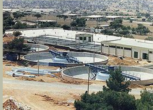
Aspropyrgos water treatment plant
