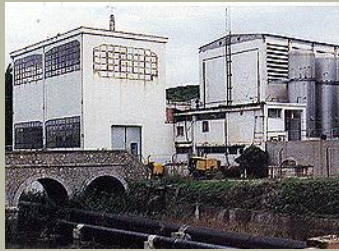
Hylike, main pumping station
