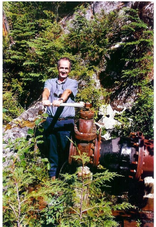
This was not surprising given the fact that the valves are operated on an closed-and-open basis; this means that they remain closed throughout the whole rainy winter season which does not enhance a smooth functioning of their mechanisms.
