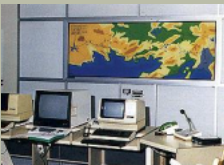
Aqueduct supervising & control centre
