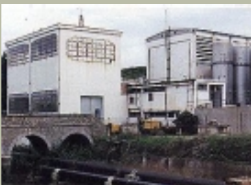
Yliki, main pumping station
