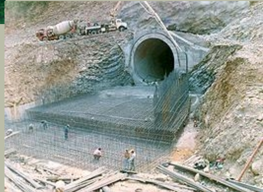
Construction of the Evinos-Mornos connection tunnel
