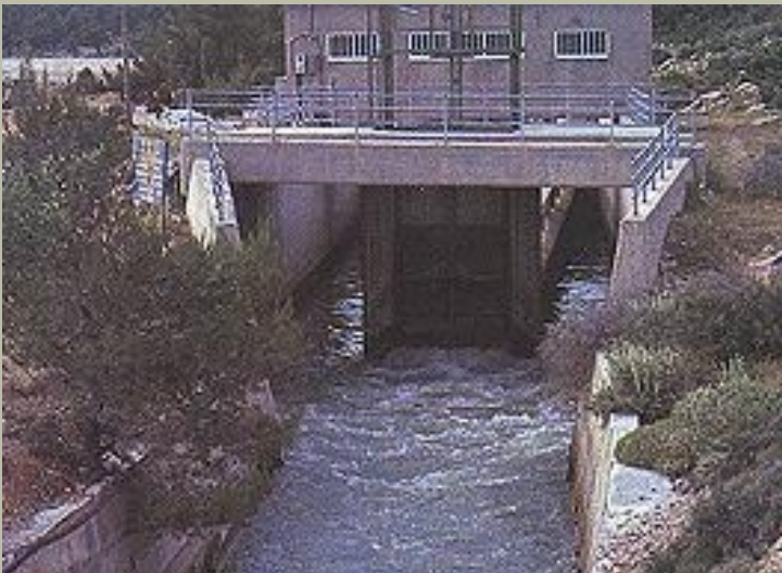
Canal flow control construction
