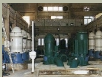
Kiourka pumping station
