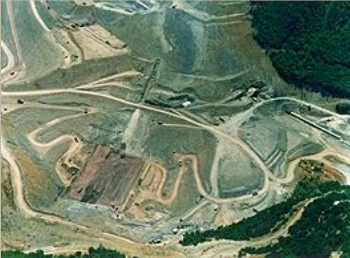
Evinos dam during construction
