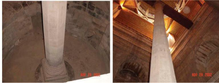
**Fig. 8** The Roda Nilometer, near Cairo, as it stands today; water entered through three tunnels and filled the Nilometer chamber up to river level (Photos: Aris Georgakakos).
