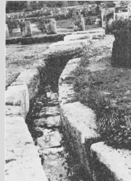
Two tributary sewers at Ceramicos (left) and agora (right) (photos from Papademos, 1975).
