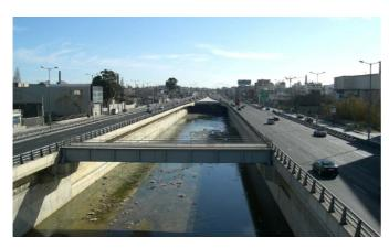
Fig. 5: Combination of the drainage channel with Kephisos Avenue (Source: Laskaris 2008)
