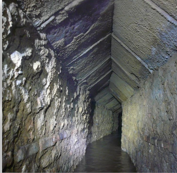
Main tunnel with inflows through the walls
