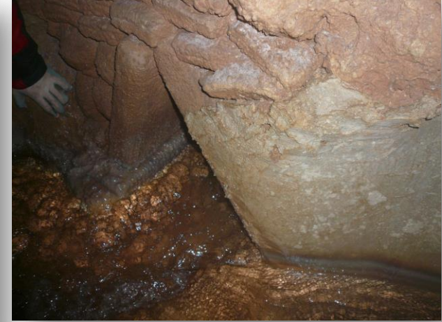
Lateral inflows through small works
