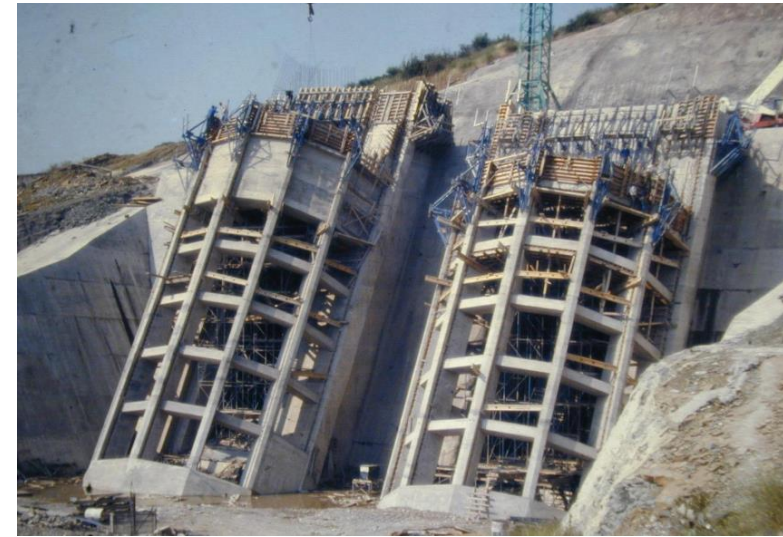
Stratos dam: inclined intakes under construction
