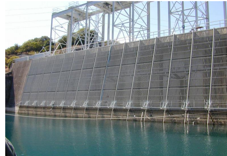
Kastraki dam: trash racks and gates
