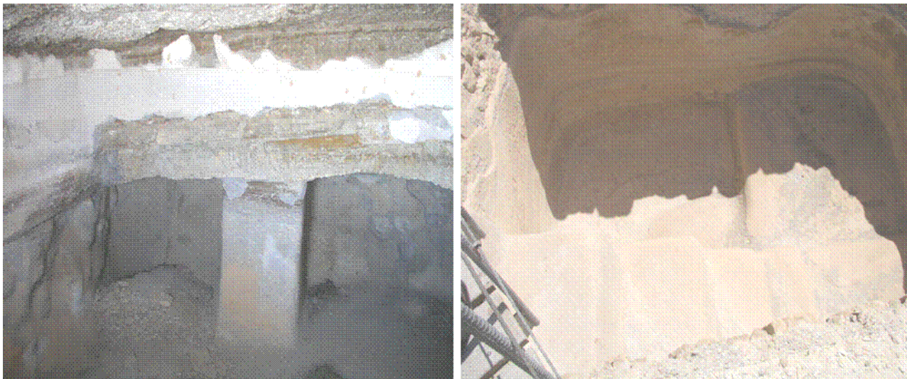
Figure 3. Water cisterns in the fortress of Masada used for harvesting and storage of rainwater.
