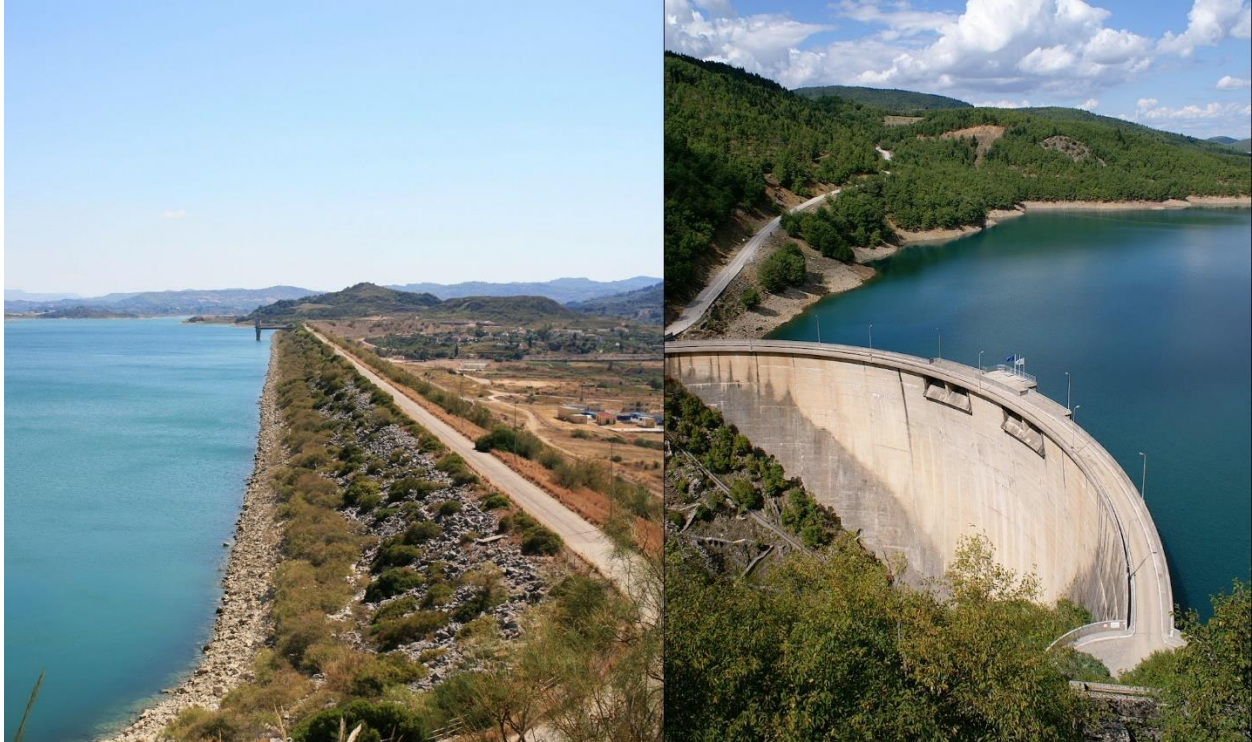
Figure 3 Photographs of Pinios (left) and Plastiras/Tavropos dam (right) 5 .
