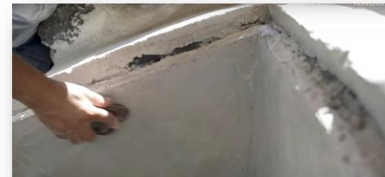
Application of last layer with Kochlidi, available in: https://www.youtube.com/watch?v=hSp40FHf8Hw&t=3s
