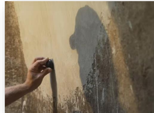
Application of last layer with Kochlidi, available in: https://www.youtube.com/watch?v=hSp40FHf8Hw&t=3s
