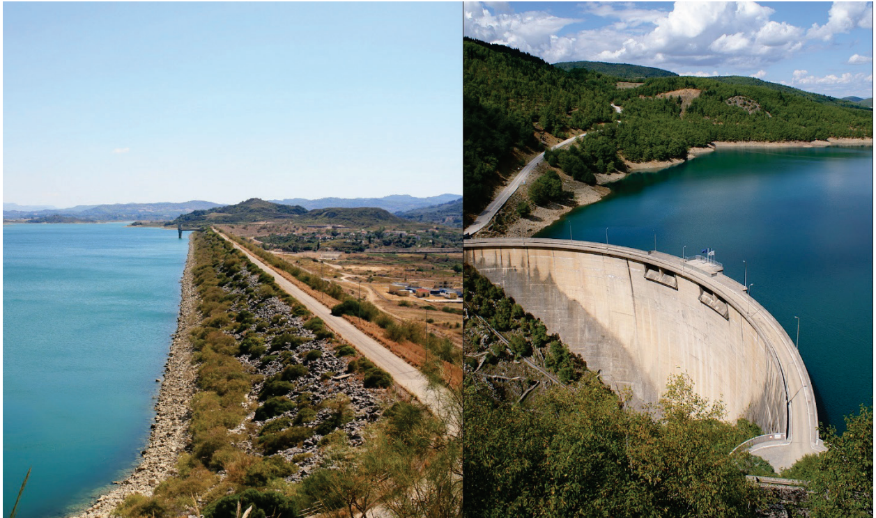
Figure 28. Photographs of Pinios (left) and Plastiras/Tavropos dam (right) 16 .
