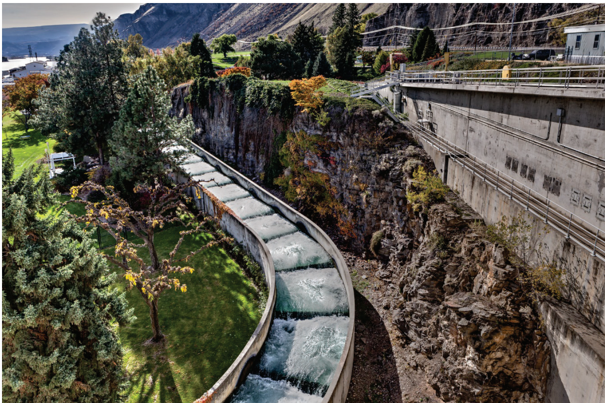
Figure 24. Example of dam with landscape design of appurtenant structure, in this case of fish pass, - Rocky Reach dam (USA). Image source: https://lh5.googleusercontent.com/p/AF1QipP518DvzPQGwTKryb0t7UbOCAK13UYkWI74 30_w=h1440
