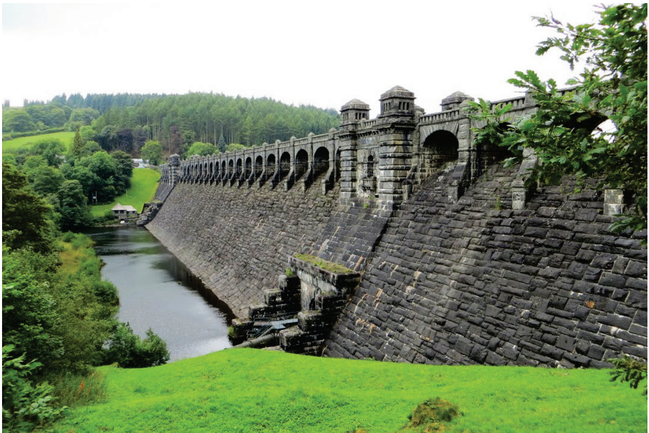
Figure 17. Example of dam with architectural intervention in downstream slope facing – Vyrnwy dam (UK). Image source: https://lh5.googleusercontent.com/p/AF1QipOcDGloGN27CJyFFeTsU9F6vz6lLeUja7CjzgO=h720
