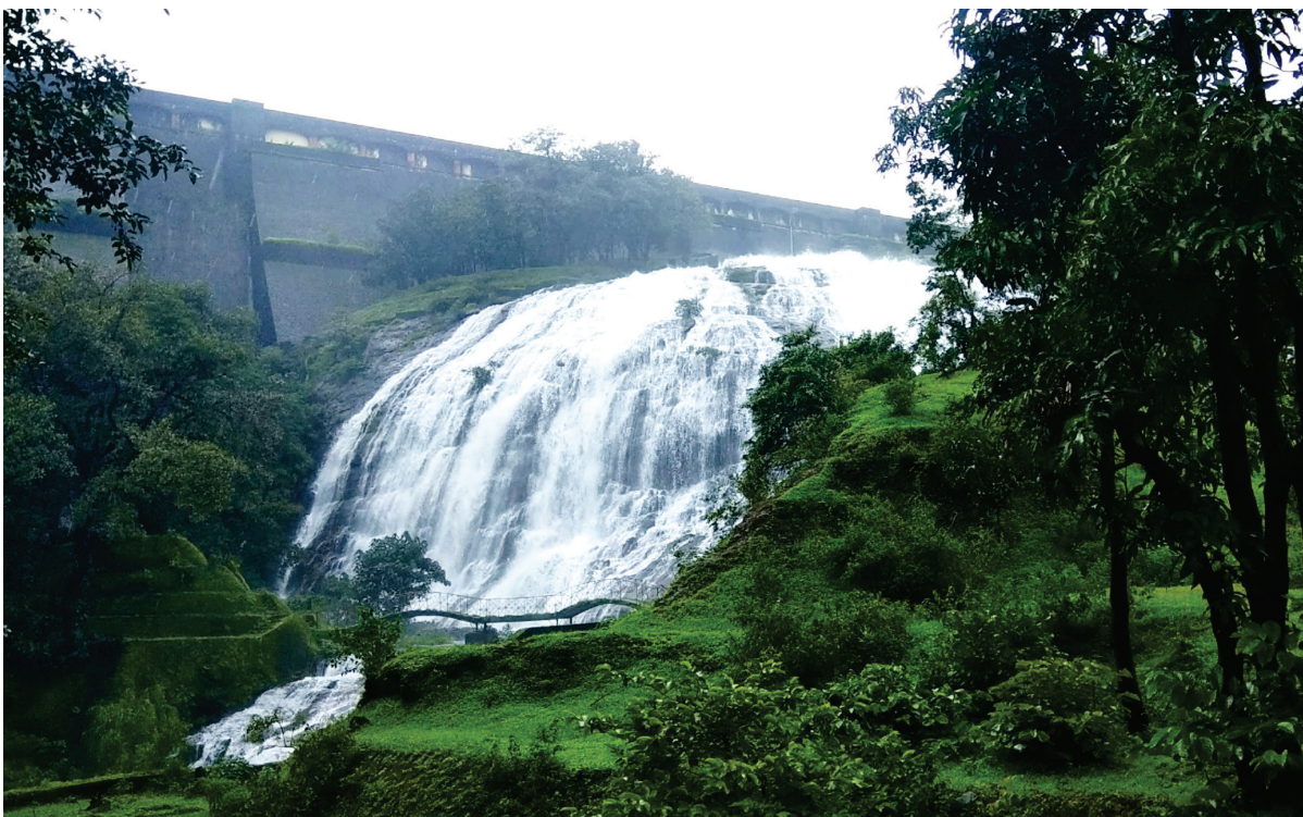
Figure 22. Example of dam with non-standard landscape design of outlet works - Bhandardara or Wilson (India) with overflow of outlet water on rocky dam abutments. Image source: https://lh5.googleusercontent.com/p/AF1QipNviWUiYR_Yu0jWixBF5irk27i0beAhEJMH6VwN=h720
