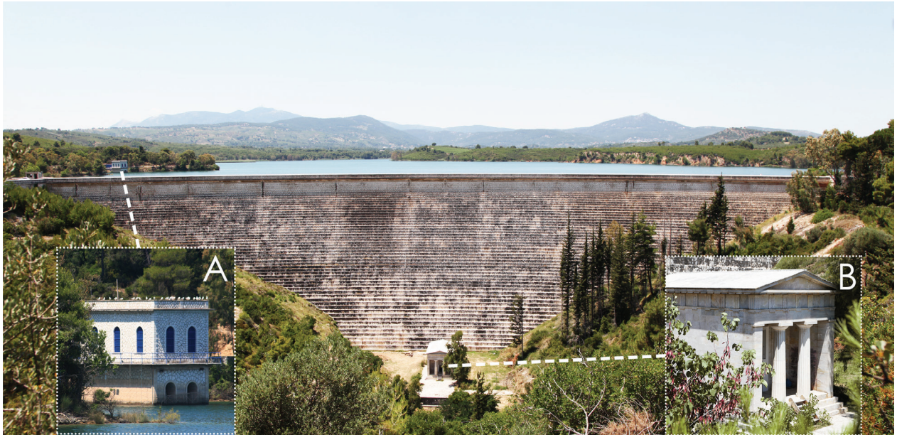
Figure 8. Example of architecturally designed dam (Marathon dam in Greece). Picture of the downstream face of the dam, which is overlaid with marble from the mine of Penteli that was also used to build the Temple of Parthenon, including pictures of architecturally designed appurtenant structures: (A) water intake tower, with similar design with the downstream face of the dam and (B) reservoir control building at the base of the dam, built to resemble the ancient temple-like structure called Thesaurus (treasure) and built after the victorious battle of Marathon (480 BCE) in Delphi. The new building was given this form in order to symbolize the victory of modern Athens in the battle against water scarcity. The dam of Marathon is not a hydroelectric dam but is indicative of the architectural adaptability of dams and their appurtenant structures, that can, and has been utilized in hundreds of hydroelectric dams internationally. Technical information on Marathon dam can be found in Soulis et al. (Soulis et al., 2019).
