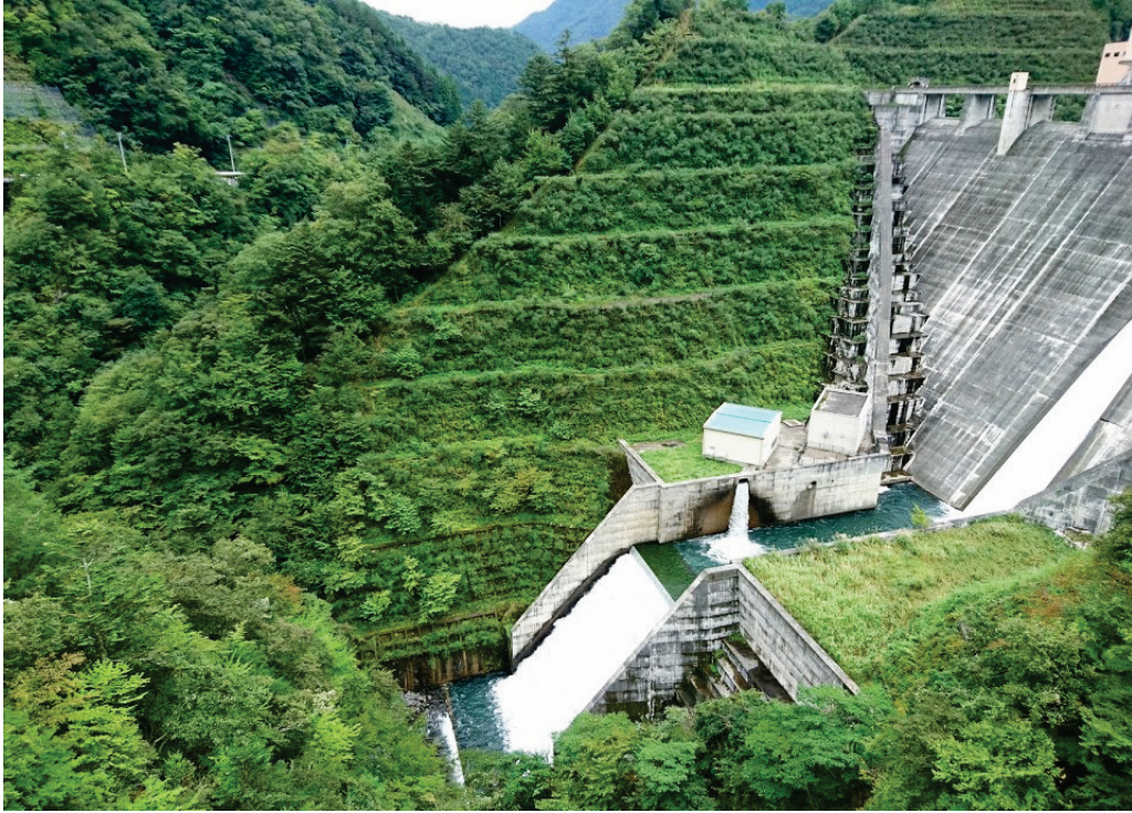
Figure 25. Example of dam with restored excavation slopes – Fukushima dam (Japan). Image source: https://lh5.googleusercontent.com/p/AF1QipN8v9YgphbIHZA_A_S2kFEMImwiksyMkRv_Ooq_=h720
