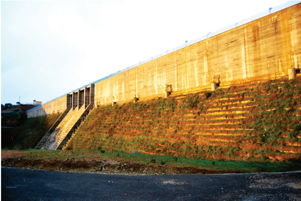
Figure 18. Example of dam with planted downstream face - La Breña II (Spain). Image source: https://lh5.googleusercontent.com/p/AF1QipM5InliGbt4FyZqMJG1GdY73tAet1oodIPGB=h1440
