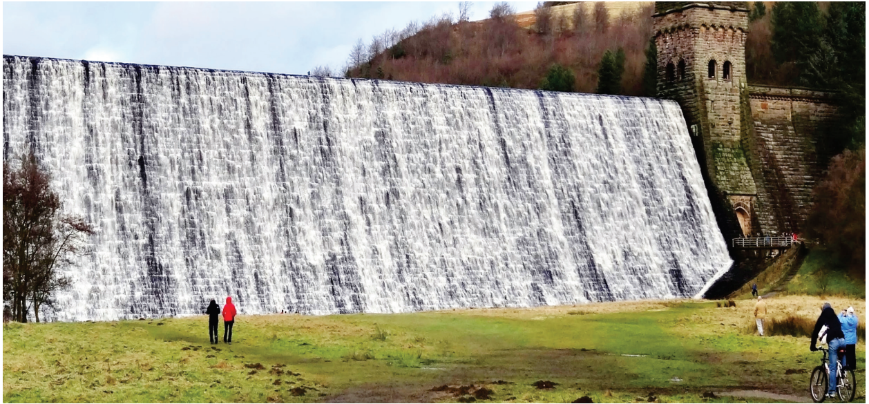
Figure 23. Example of dam with a special architectural design of its spillway with overflow over dam body – Derwent dam (UK). Image source: https://lh5.googleusercontent.com/p/AF1QipNV_vl6wBhjacDsGQLuWEC EL2h-UkFP7v_3Mc2E=w1280-h720-pd
