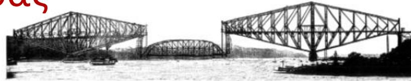
Figure 10. The span linked to the chains and raised clear of the scows, attempting the last hazardous operation in the construction of the bridge.
