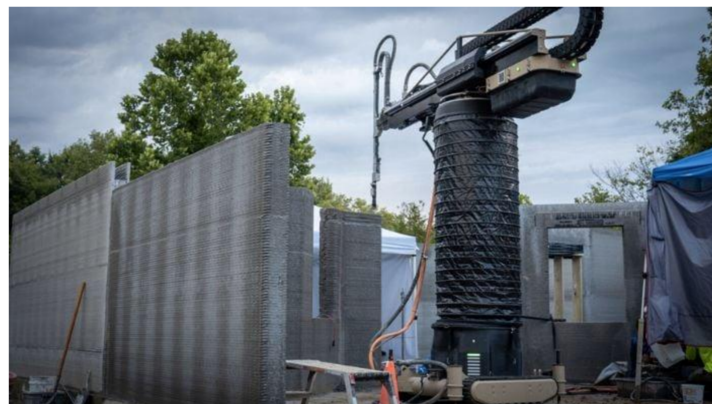
β. Apis Cor (American company from Melbourne) printer with nicknamed 'Frank'.
