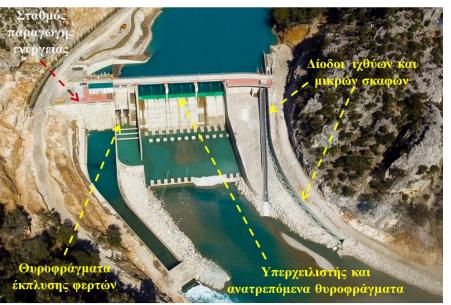
2 turbines Kaplan S-Type, power 5.93 MW (5-40 m<sup>3</sup>/s) Mean annual electric energy production 40 GWh
