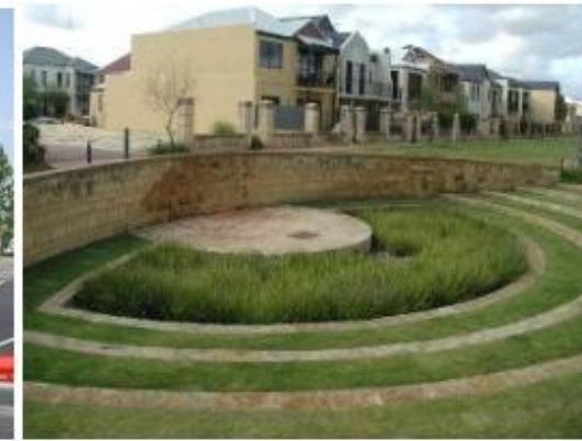
Bioretention in Perth
