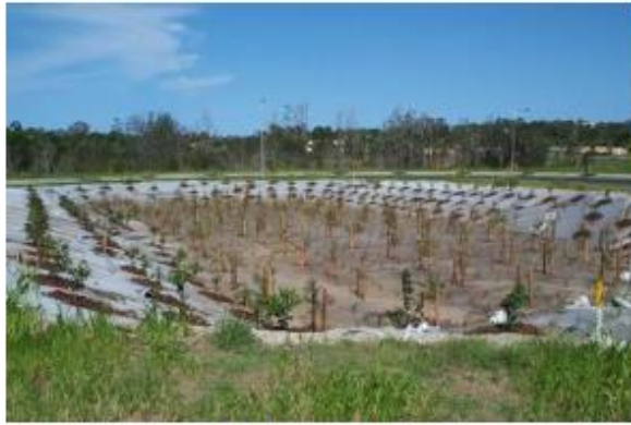
Blacken Ridge Bioretention Basin (BCC)
