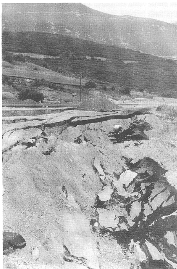
Fig.9.8. Failure of road embankment with poor foundations on weathered flysch and lacking drainage
