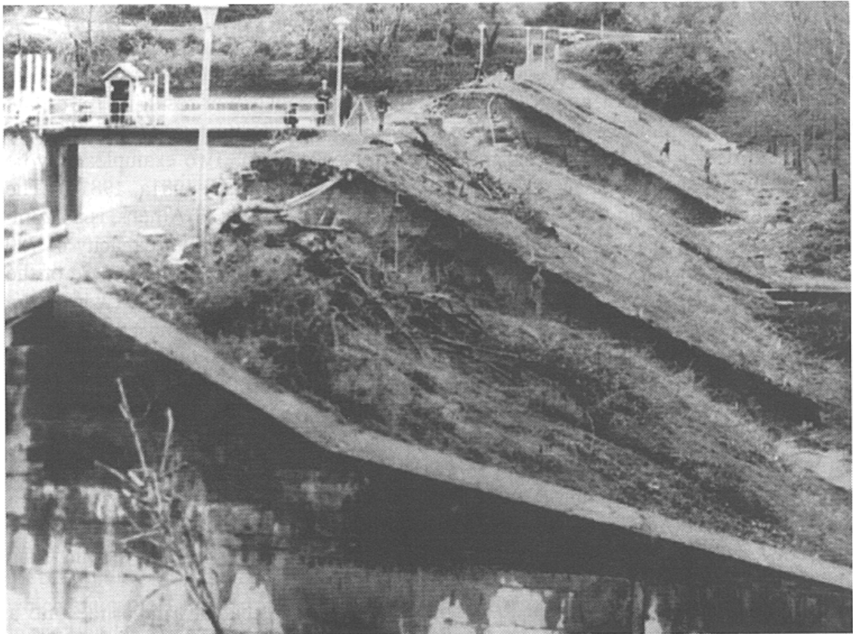
Fig.9.16. A view of the breaches in the Agras dam caused by the flood of 18-19 November 1979
