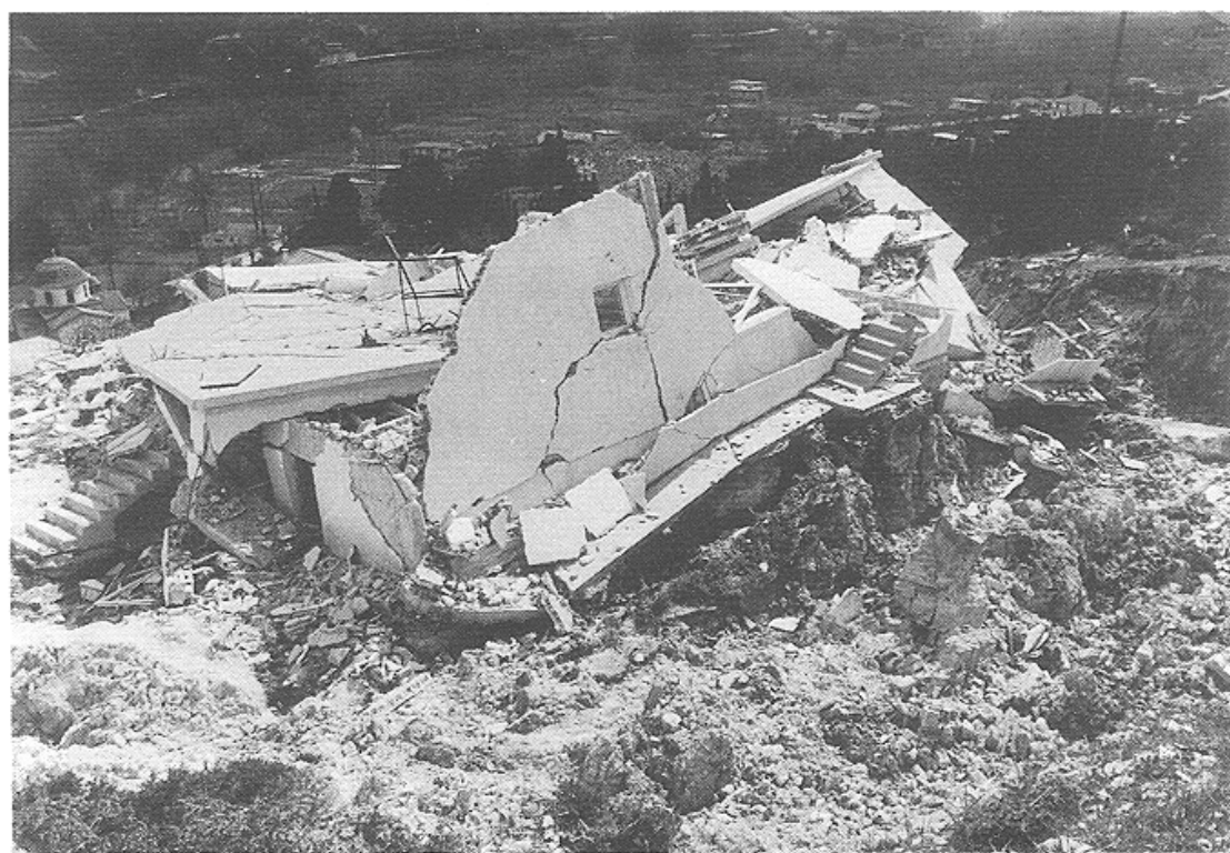
Fig.9.7.A ( upper ): Rotational slides in marly Neogene sediments, transformed into earthflows near the foot which abut on the Preveza-Igoumenitsa road, western Greece. B ( lower ): Collapsed house built on clayey-marly Neogene sediments
