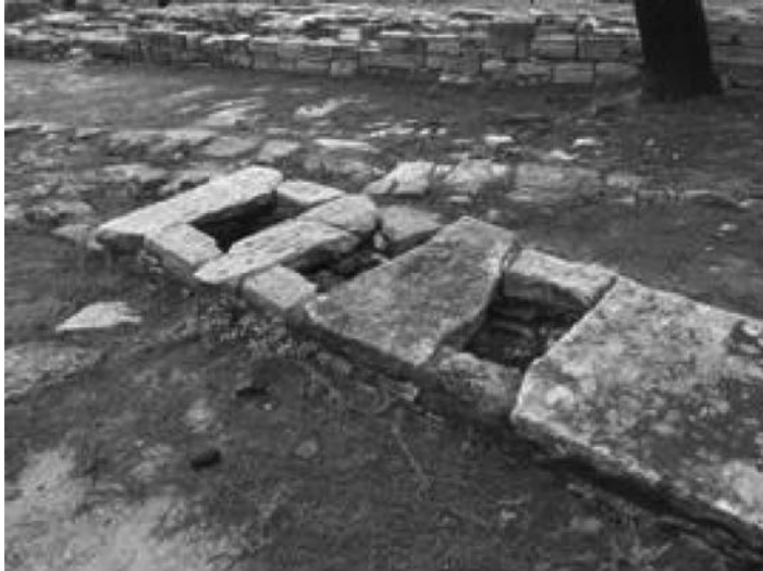
Figure 14.2 Minoan aqueduct in Tylisso, Crete, brings water from springs (with permission of L. W. Mays)
