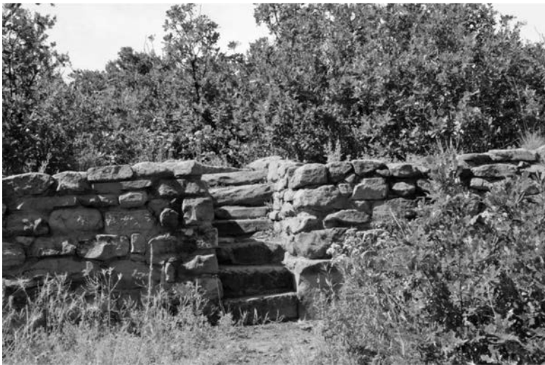
Figure 15.7 Restored stairway at Far View Reservoir in Mesa Verde National Park. Stairway not only functioned as a way to reach the stored water but also may have had special social or religious function (with permission of L.W. Mays)
