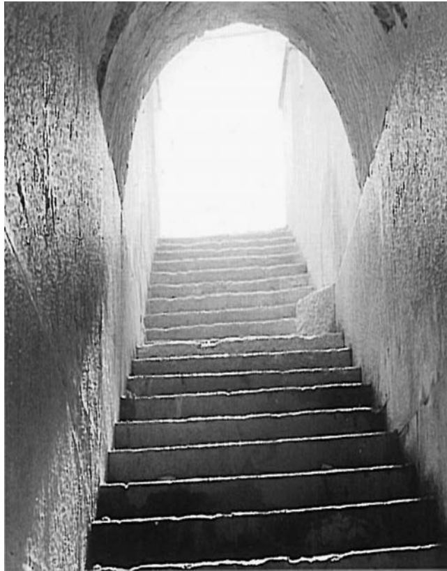
Figure 5.16 Access way to the sewerage networks
