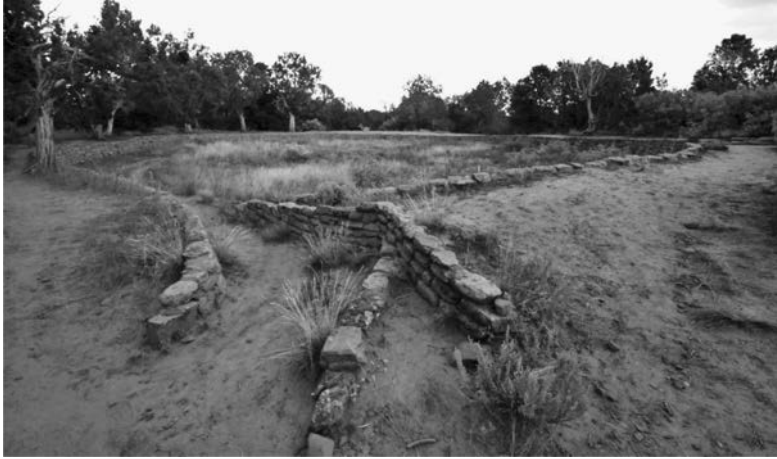
Figure 15.6 Far View Reservoir at Mesa Verde National Park. In the foreground is the restored intake structure (canal) into the reservoir (with permission of L.W. Mays)
