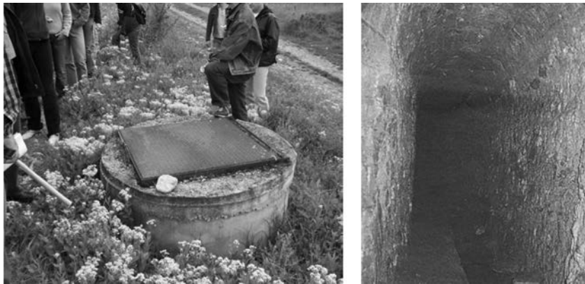
Figure 4.10 Left: The initial well (shaft) of a qanat in Nea Zichni (with permission of K. Voudouris). Right: The tunnel of a qanat at Chortiati, Thessaloniki constructed in the 18th century (with permission of K. Voudouris)
