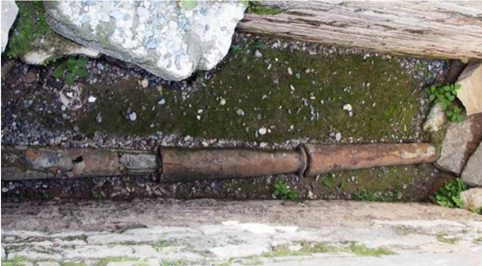
Figure 2 Aqueduct of terracotta pipes in Knossos (Angelakis et al. 2012).
