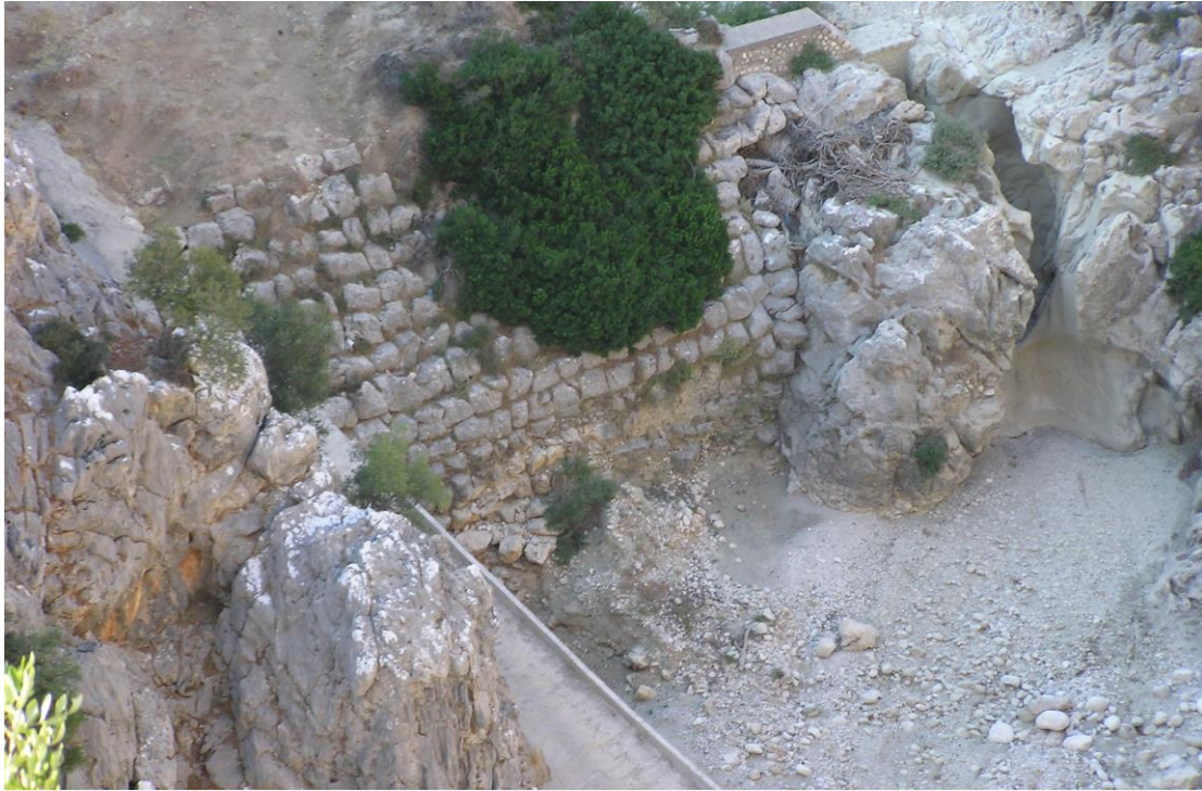
Figure 8 The Alyzia dam in Western Greece. On the right the spillway with its irregular shape formed by erosion through centuries; the photo was taken in summer, when the stream has no water (courtesy of N. Zarkadoulas).
