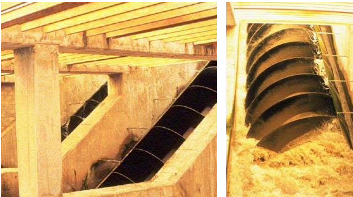
Figure 10 (Left) A series of Archimedes's water screws in their modern form (in which the walls are not attached to the screw), as implemented in the wastewater treatment plant of Athens, which pump 1 million m 3 of wastewater per day. (Right) Detail showing one helix.
